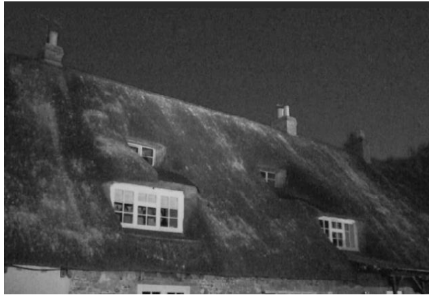
Figure 2: Screenshot for camera at northern elevation
