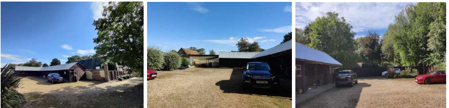
Figures 93 – 95 Views of gravel parking area & access track and modern stables.
