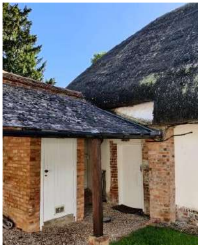
Figure 84 Furthest bay – 1997 extension incorporated 1890s single storey extension with thatch roof. 20 th century slate roof lean-to with 1997 boiler cupboard.
