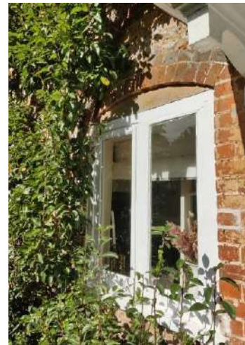
Figure 68 early 19 th century brick and flintwork bands with brick quoins.
