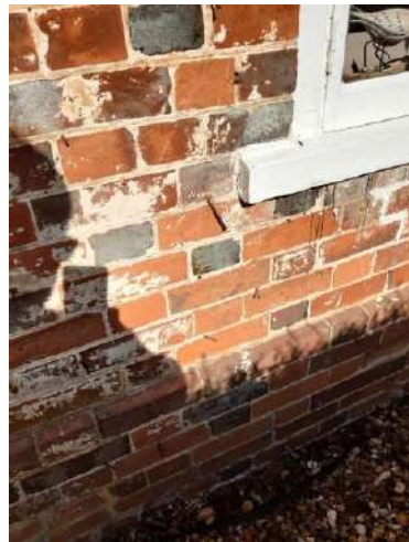
Figure 68 early 19 th century brick and flintwork bands with brick quoins.
