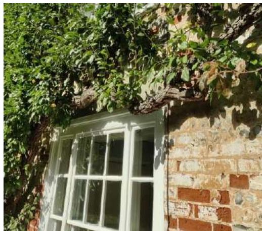
Figure 71 early 18 th century flinwork walls with brick quoins with sash windows and six panel door with pediment surround.
