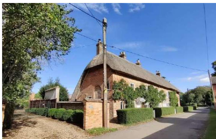
Figure 1 View of south and west elevation from Newbury Hill
