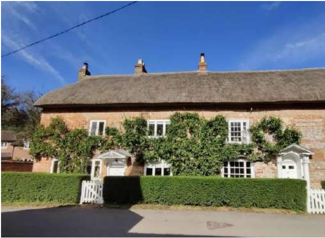
Figures 40 & 41 Front (south) elevation showing brick and knapped flint bands.
