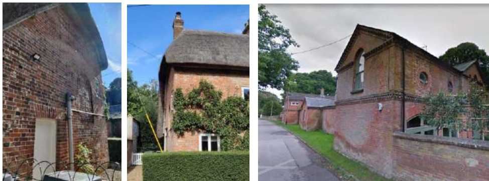
Figures 50 & 51 West end of property showing areas of 19 th brickwork refacing Figure 52 Google maps image of adjacent stable block (now converted to homes and nursery).
