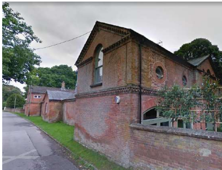
Figure 79 Google maps image of adjacent stable block (now converted to homes and nursery).
