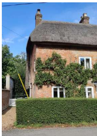
Figure 67 Mid 19 th century (approx. 1865) brick refacing – far left of south elevation
