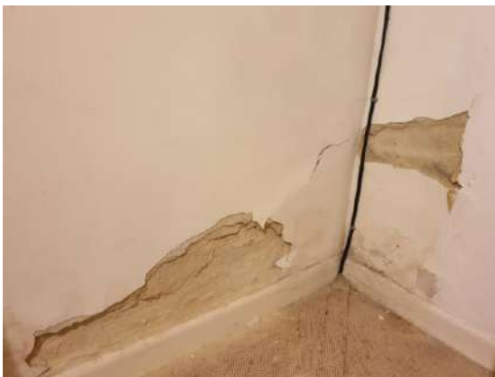
Figure 140 Damaged plaster in Games Room Figure 141 Cracking in north wall of Dining Room Figure 142 Crumbling and cracking of ceiling above staircase
