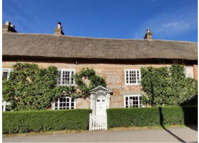
Figures 40 & 41 Front (south) elevation showing brick and knapped flint bands.
