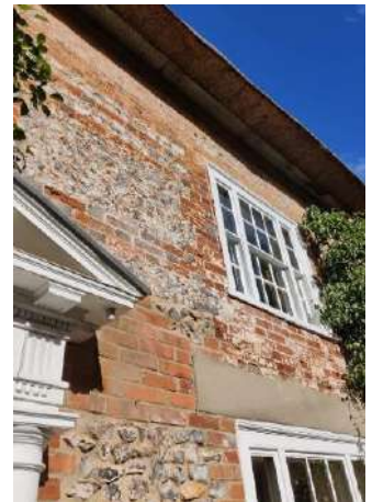
Figure 71 early 18 th century flinwork walls with brick quoins with sash windows and six panel door with pediment surround.
