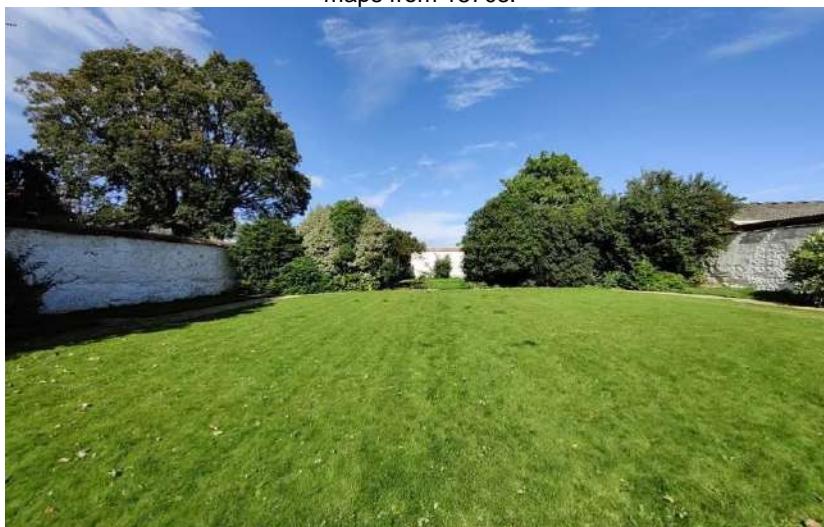
Figure 8 View towards back of garden showing historic boundary wall
