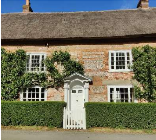
Figure 71 early 18 th century flinwork walls with brick quoins with sash windows and six panel door with pediment surround.
