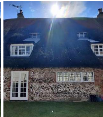
Figure 84 Furthest bay – 1997 extension incorporated 1890s single storey extension with thatch roof. 20 th century slate roof lean-to with 1997 boiler cupboard.
