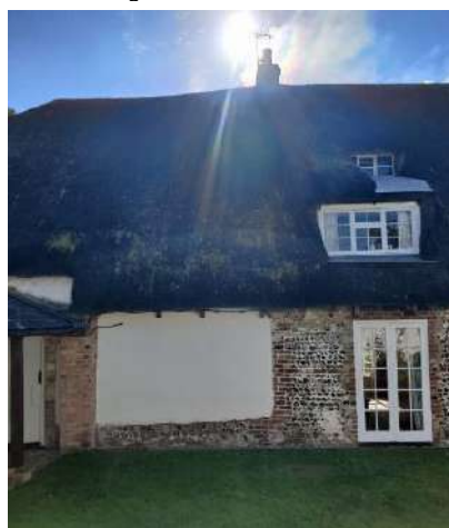
Figure 84 Furthest bay – 1997 extension incorporated 1890s single storey extension with thatch roof. 20 th century slate roof lean-to with 1997 boiler cupboard.
