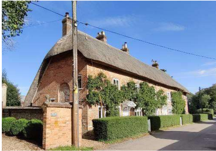
Figure 107 Views of south (front) gravel areas bounded by Newbury Hill.
