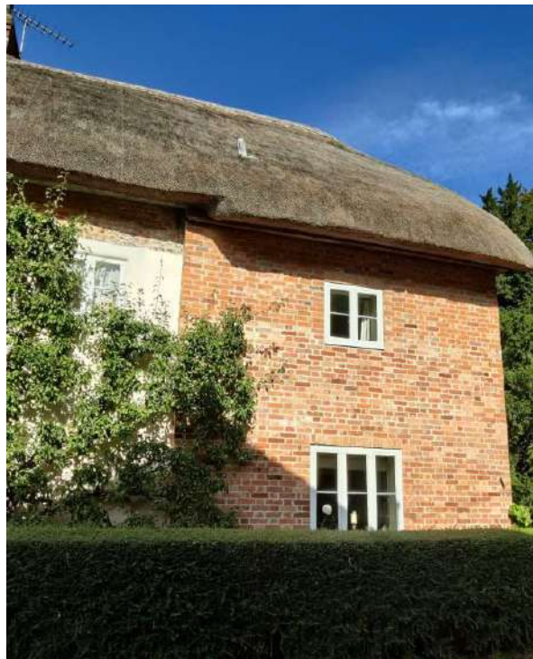
Figure 74 Early 19 th century rendered bay and 1997 brick extension.
