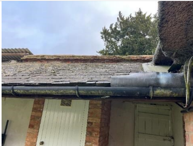
Although there are gaps within the roof structure, it is not lined and unsuited for bat roosting
