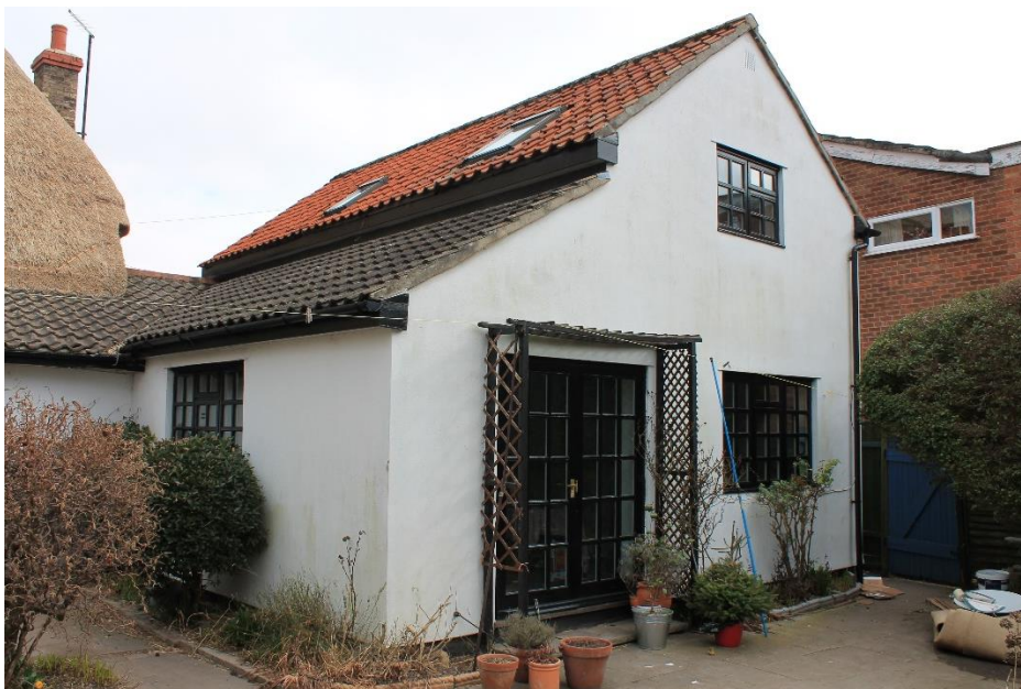
Photograph 6: windows to 1990s rear extension
