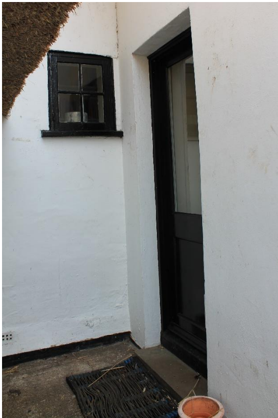
Photograph 3: existing external door to be blocked up.
