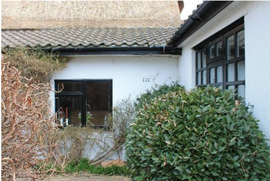
Photograph 5: window to proposed new bathroom (left) and to kitchen-diner (right)
