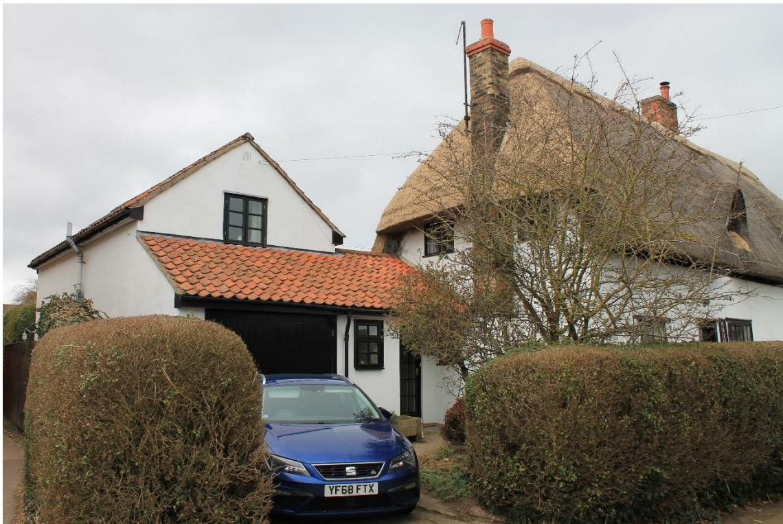
Photograph 1: front of property from Lode Road
