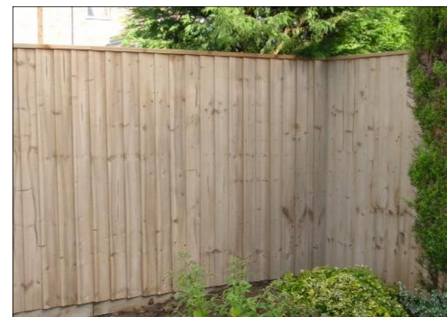
Close boarded fence along the sides and rear boundaries
