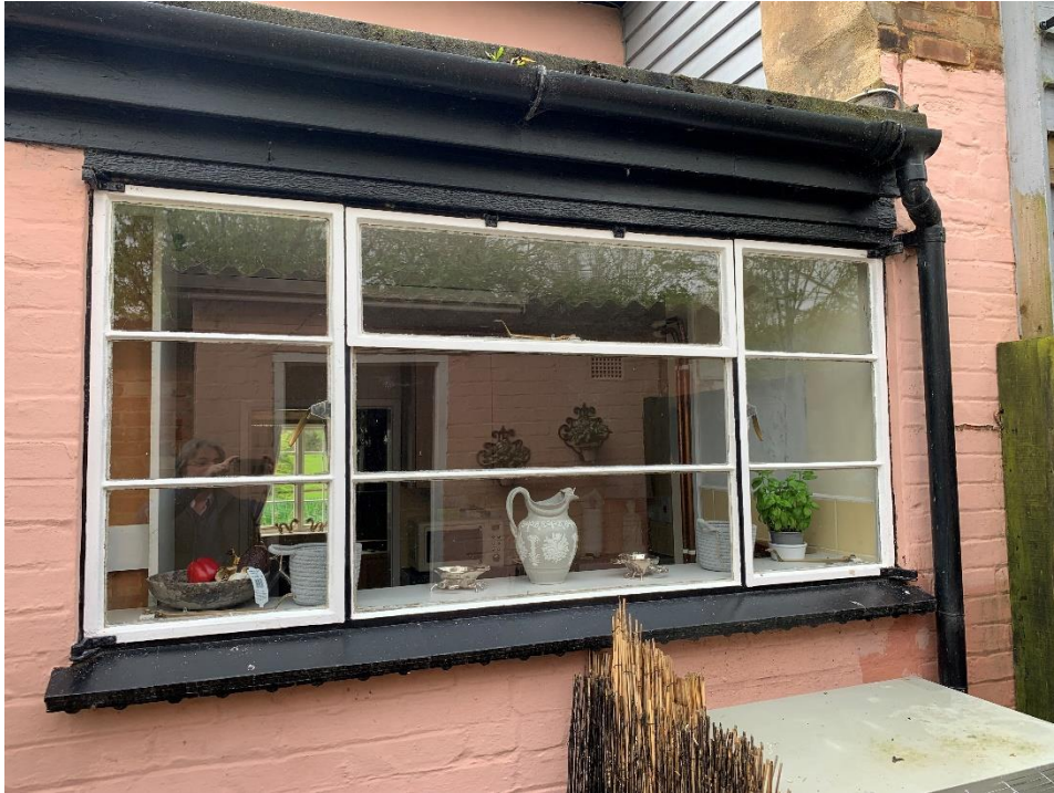
Metal framed and single glazed with creasing tile cill
