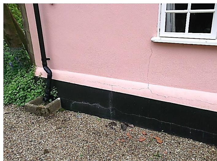
The image left shows typical cracking to the cementitious render.
