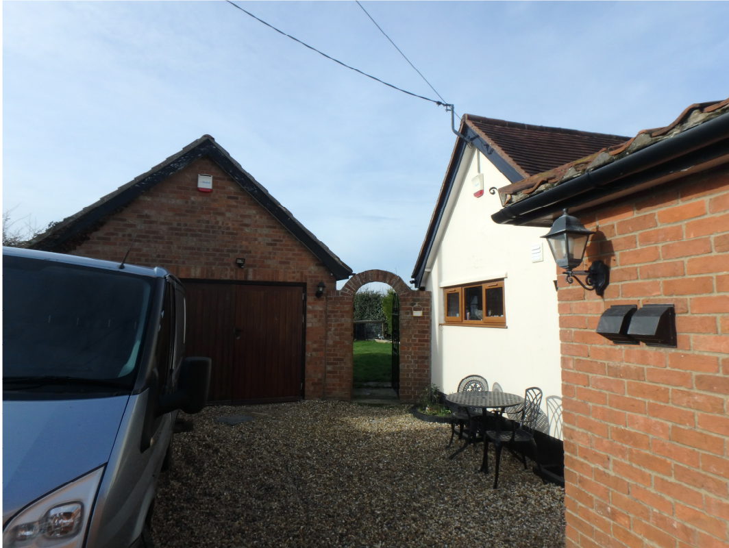
View showing side elevation of existing rear extension connected to the existing detached garage by a brick wall and solid gate, these will obscure the view of the proposed extension from the front and side
