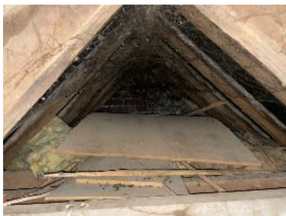
Plate 5: Internal roof space
