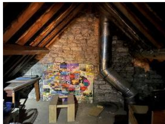
Plate 4: Internal roof space
