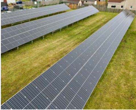
Fig 6) Example of a completed installation
