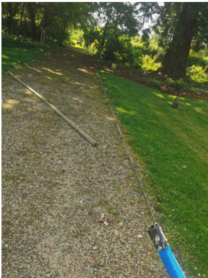
Fig 9) Proposed route of excavation through the grounds of Mendlesham Manor
