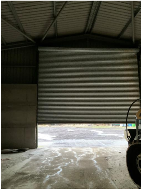
5. Front of Grain Barn from inside. Note diagonal bracing in roof.
