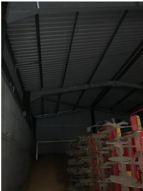
7. Roof - Steel purlins at wide centres spanning between steel frames.
