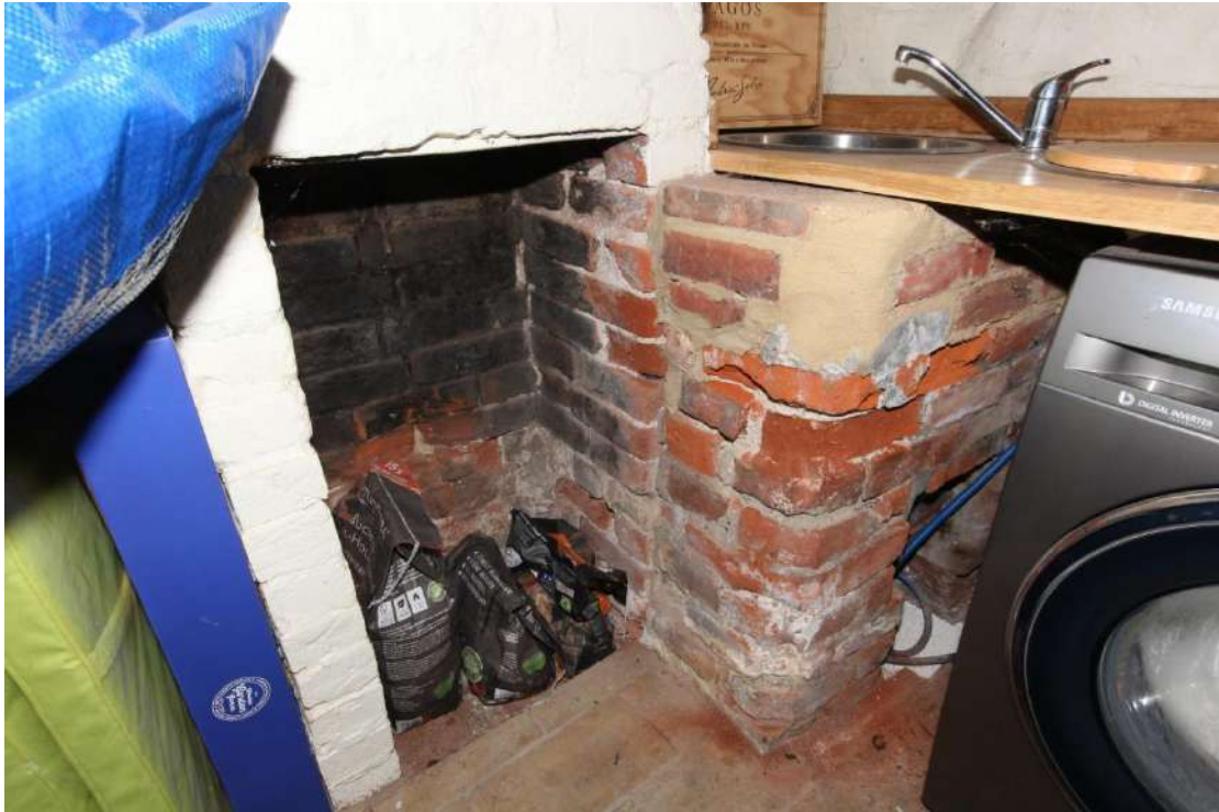
Illus. 5. A detail of the fireplace in illustration 4 with the stoke-hole of the brick copper base visible to the right. The copper was presumably a slightly later addition as its brickwork is not integral to that of the main chimney. The position of the copper itself is hidden by the modern work top but it is understood to have been removed.
