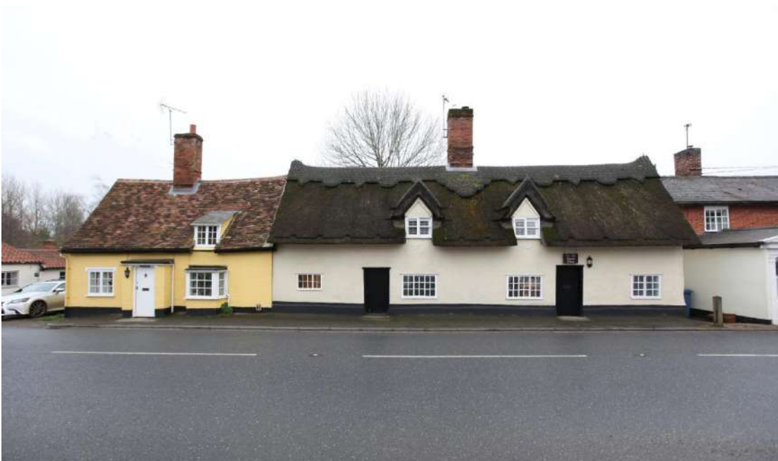
Illus. 2. The Old Thatched Cottage was built as two almost mirror-image tenements and retains its original symmetrical facade with twin entrance doors – although the door on the left is blocked. The property shares a single listing entry with its earlier tiled neighbour to the left. The unusual, projecting single-storied 19 th century structure on the right is understood to have operated most recently as a tailor's shop.
