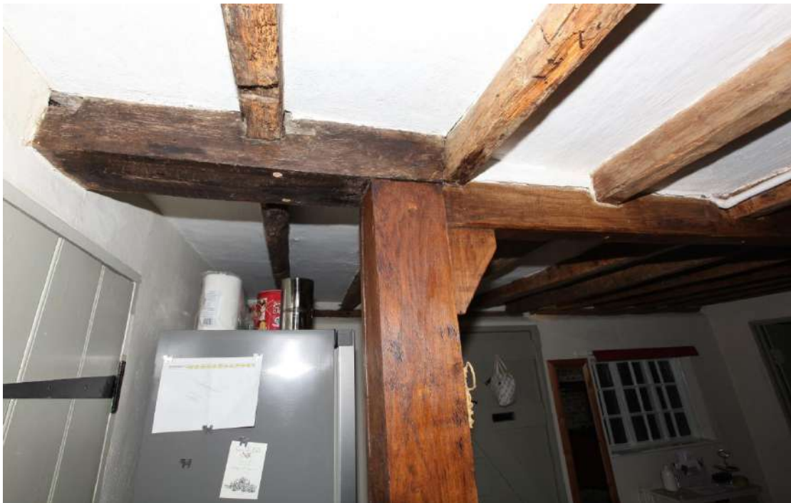
Illus. 18. A detail from the rear of the modern post which supports the two axial ceiling joists in the western cottage. The same task was originally performed by a studwork partition matching that in illustration 13, the notches of which are visible in the common joist immediately above. The common joists are all re-used, retaining nails, mortices and notches from their former lives, but those to the left are tenoned to a substantial axial joist while those on the right span the building and are supported by a narrow length of pine in the centre. The pine has been abraded and cleaned to the west of the chimney, producing a modern appearance, but preserves its original surface on the east.
