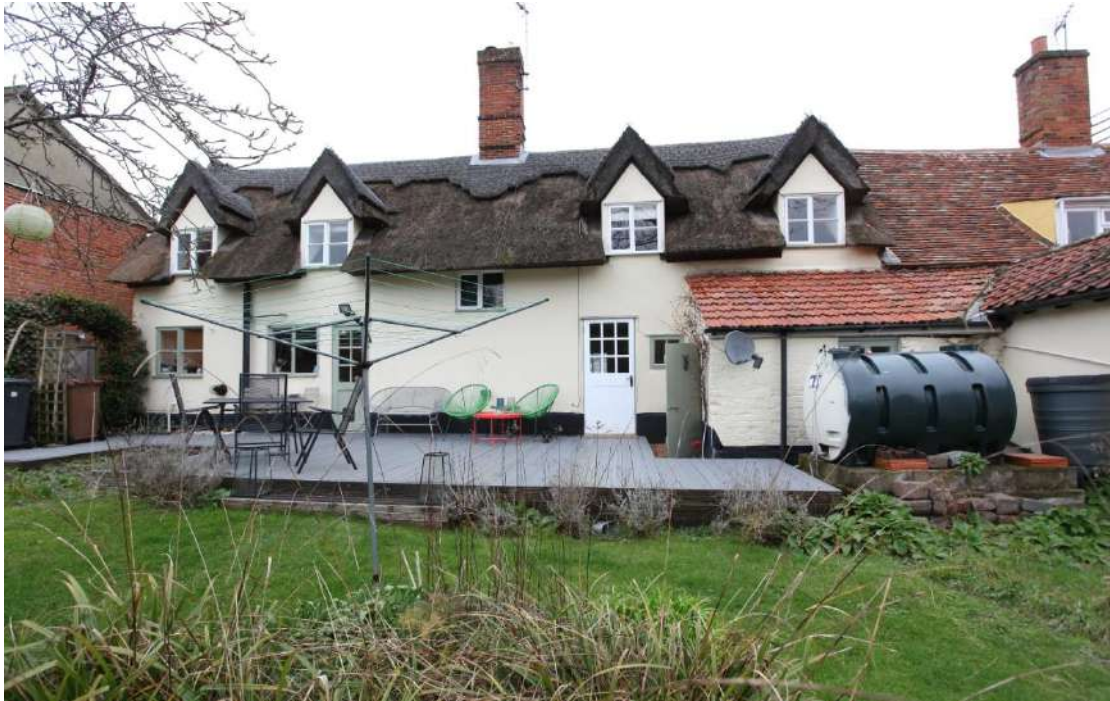
Illus. 3. The still largely symmetrical rear elevation with the brick and pantiled mid-19 th century lean-to addition on the right. Built as a wash-house its original external chimney has been removed. The unusually narrow back door of the western cottage on the left was truncated to accommodate the modern stair behind the chimney, which is longer and therefore less steep than its predecessor. Figure 9 suggests the ground-floor window to the extreme left is a later insertion, but all four dormers are original.
