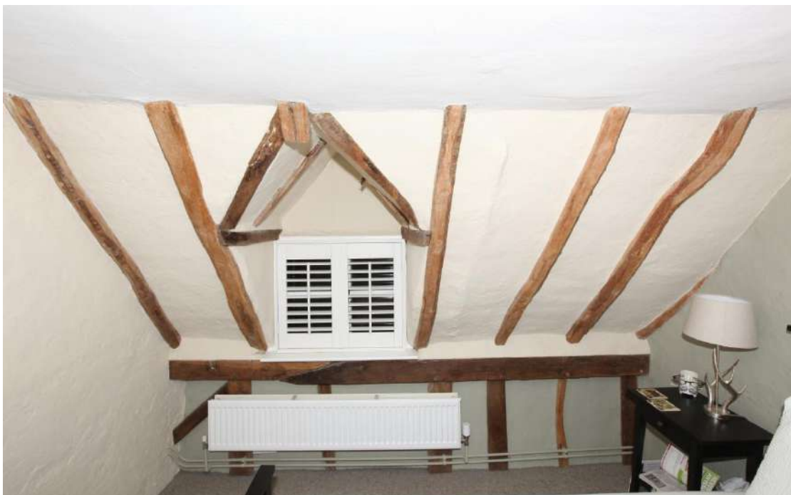
Illus. 22. The front (northern) wall of the bedroom above the living room in the eastern cottage with the original partition against the chimney and western cottage to the left. The rafters consist of slender branches with waney edges that retain much of their bark. The wall timbers, in contrast, are largely re-used from older structures and are more substantial, although some studs such as the thin example to the right are similar to the rafters (and are not re-used). The timbers of the six dormer windows all appear to be contemporary with the building.
