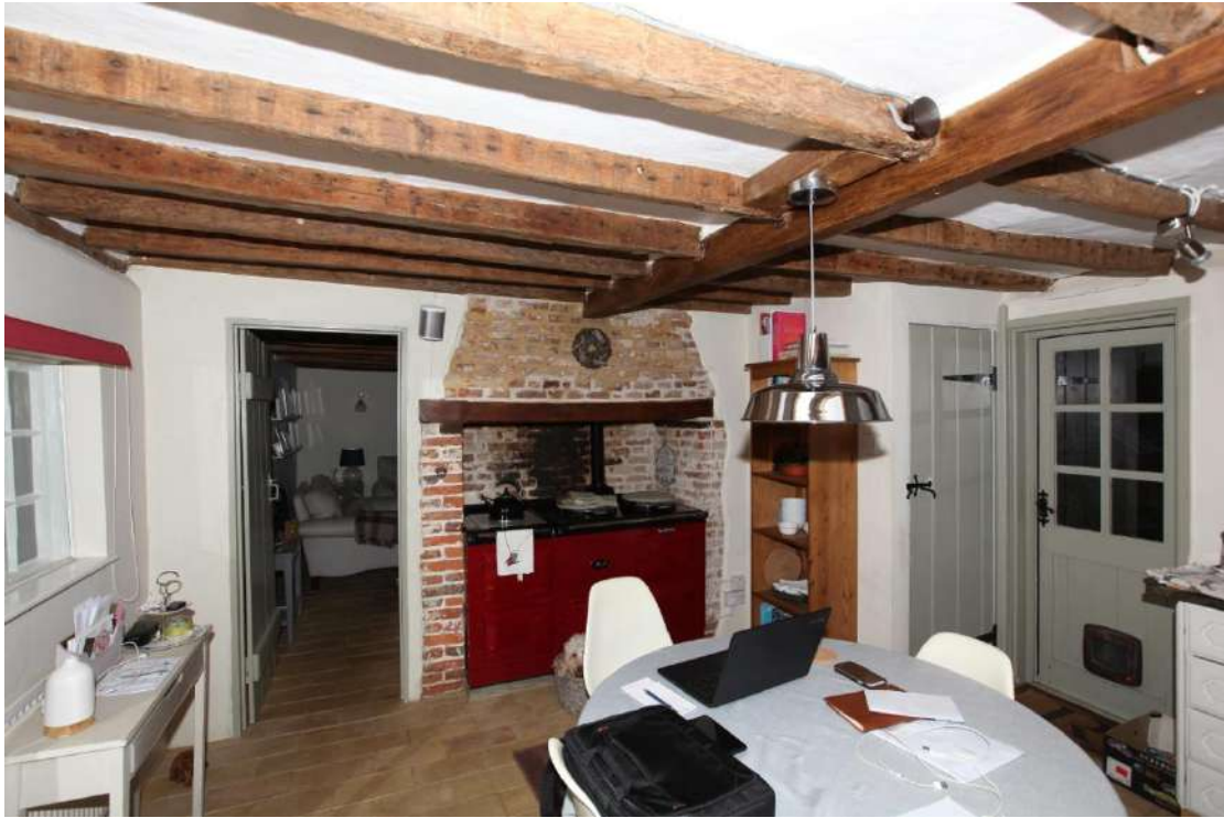
Illus. 15. The original fireplace in the hall/kitchen of the western cottage, matching its counterpart to the east. The unusual ceiling also matches, with re-used joists displaying the scars of lath-and-plaster on their sides. The cupboard-like projection on the right conceals the modern stair which occupies the same position as its predecessor but projects further into the room - hence the narrow width of the modern back door.
