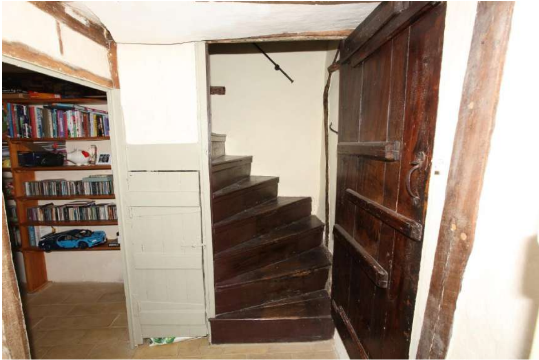
Illus. 11. The corner stair of the eastern cottage which appears to be entirely original to the building, with the re-used plank-and-batten door on the right. A similar stair lay behind the central chimney initially, but has since been rebuilt with a less precipitous incline.
