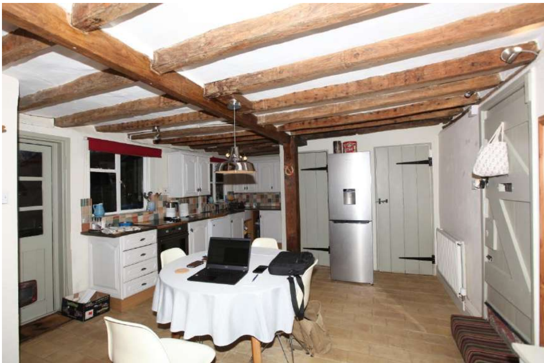
Illus. 16. The modern kitchen in the western cottage, with the original entrance door on the right. The vertical post marks the position of the missing partition between the hall and pantry – and the two ceiling structures. The present pantry and WC partitions in the rear are modern insertions of brick or block-work and plasterboard.
