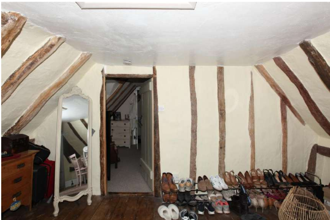
Illus. 26. The original partition of the eastern cottage, as seen from the east, showing its exposed studwork and the original connecting doorway to the western bedroom of the same cottage. The two first-floor partitions did not lie above the pantry walls on the lower storey but were placed centrally to create bedrooms of equal size.
