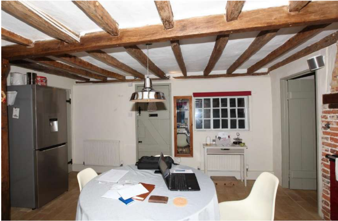
Illus. 17. The front wall of the western cottage showing its original entrance and window positions. The site of the missing western wall is indicated by the post on the left
