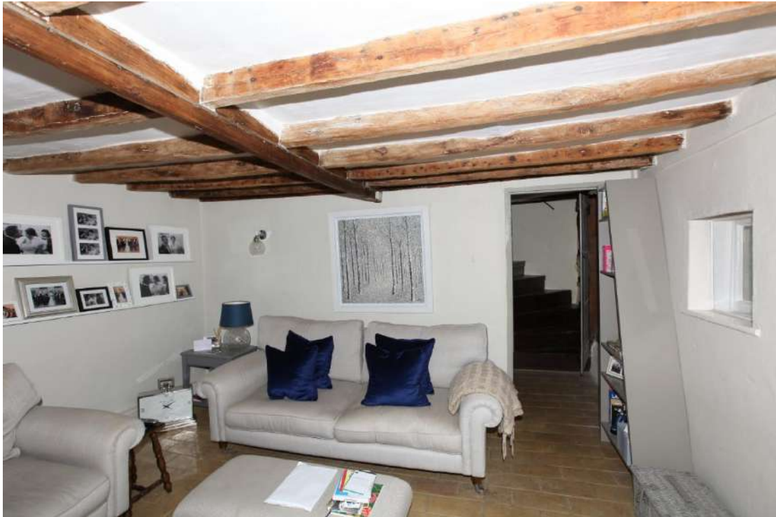
Illus. 7. The living room from the west showing the original partition of the pantry with a door to the corner stair on the right. The pantry door lay to the left but is now blocked (illus. 12), as is the front door in the northern facade to the extreme left.
