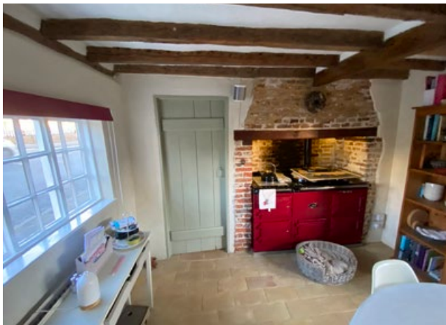
Modern wall between chimney and external wall to be removed.
