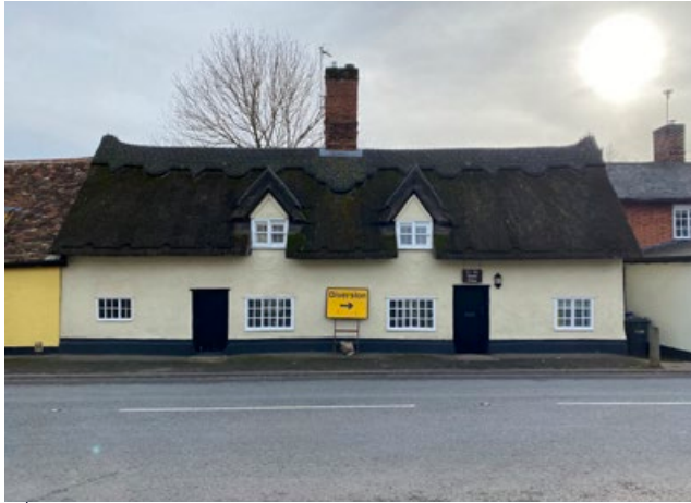
▲ Front elevation to remain unchanged in scale. First floor windows are proposed to be replaced with slimite glazed units.
