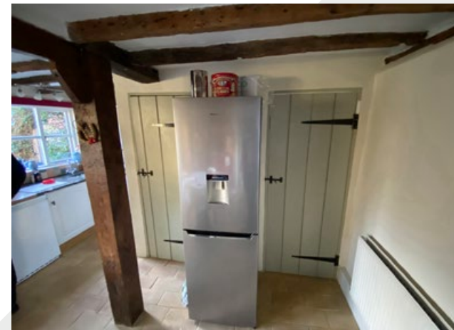
Modern internal partitions for existing WC and pantry to be removed. Downstairs WC to be relocated.
