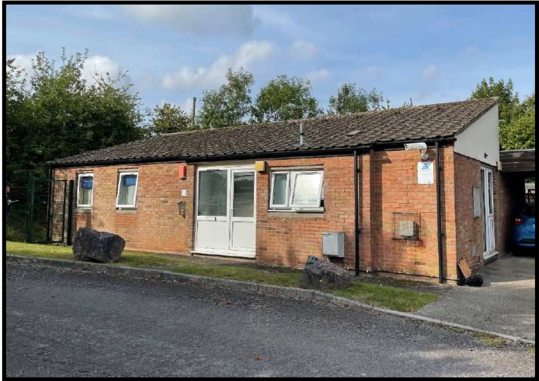
Fig. 1 - The existing caretaker's bungalow at St. Katherines Secondary School
