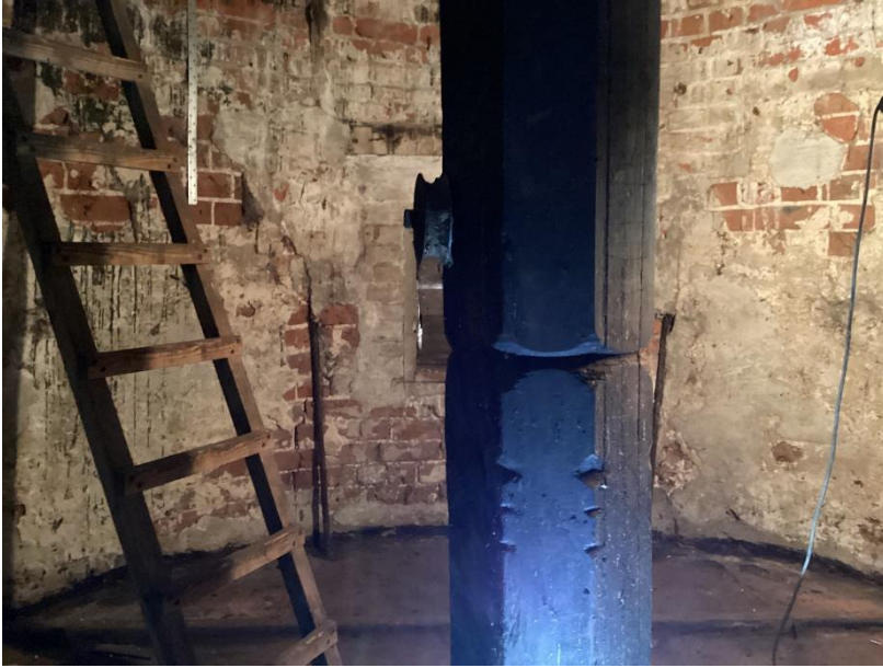
Plate 3: Building 1, interior of roof
