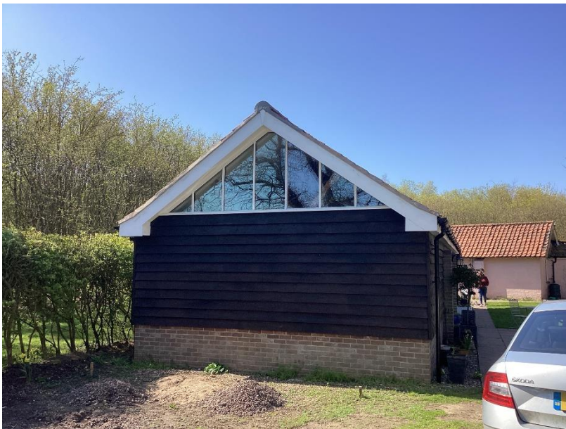
Plate 8: Building 3, north aspect
