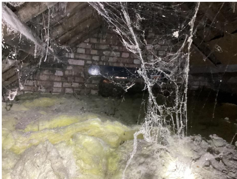
Plate 6: Building 2, roof void
