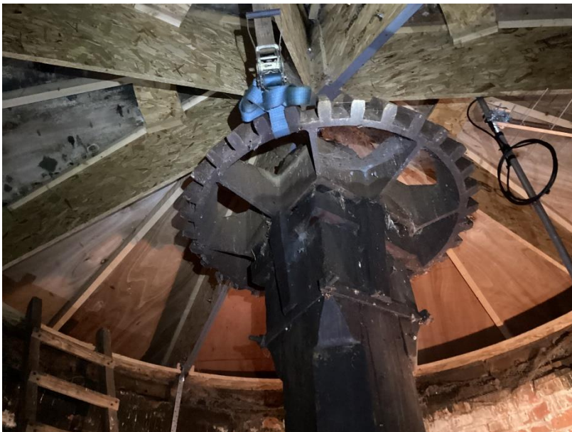
Plate 2: Building 1, interior of roof
