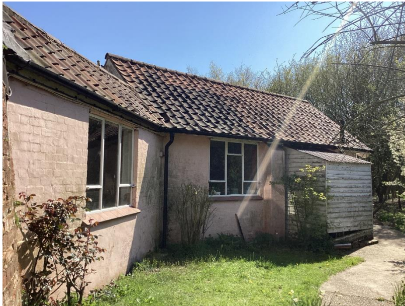
Plate 4: Building 2, south aspect
