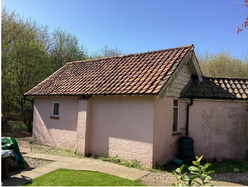
Plate 5: Building 2, north aspect
