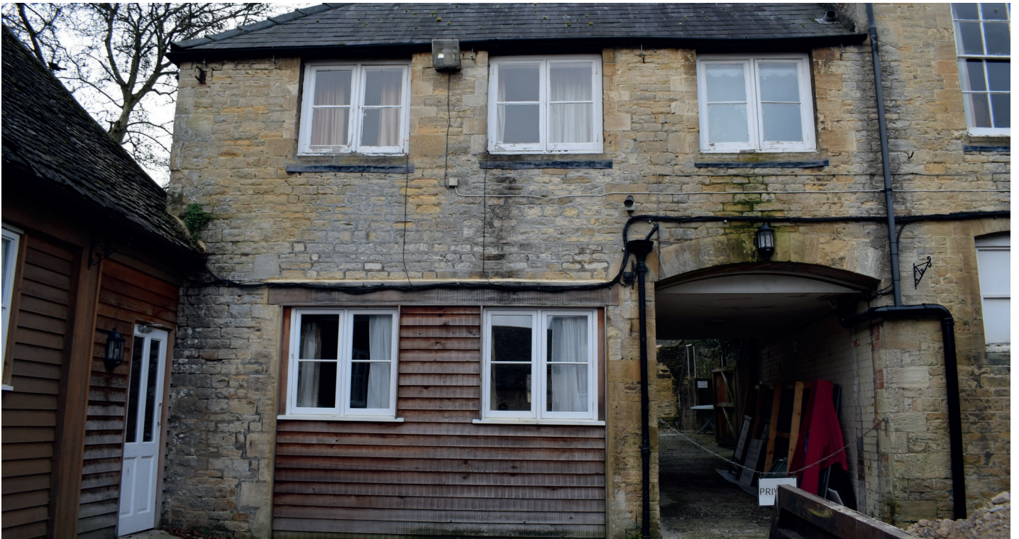
Timber cladding to be replaced with render
