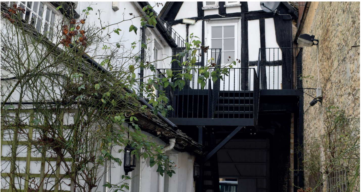
Modern timber door to be replaced with a window following removal of the external fire escape
