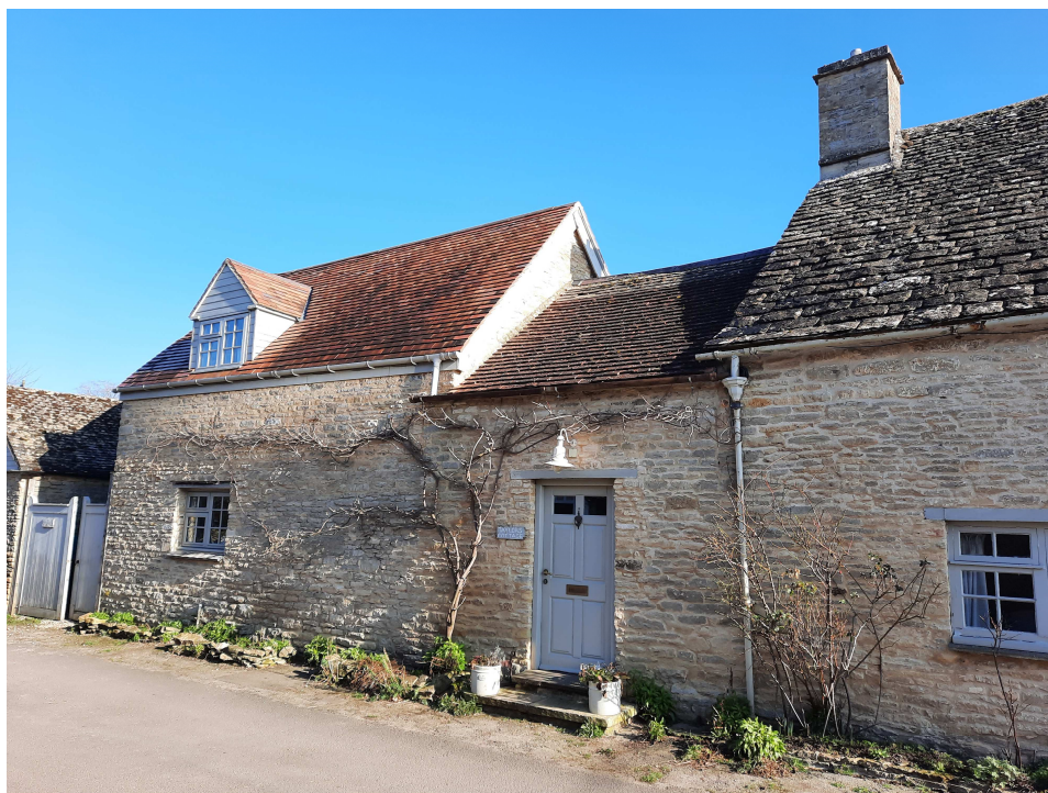
Fig 3. Part front elevation with original cottage to the right and more modern extension to the left
