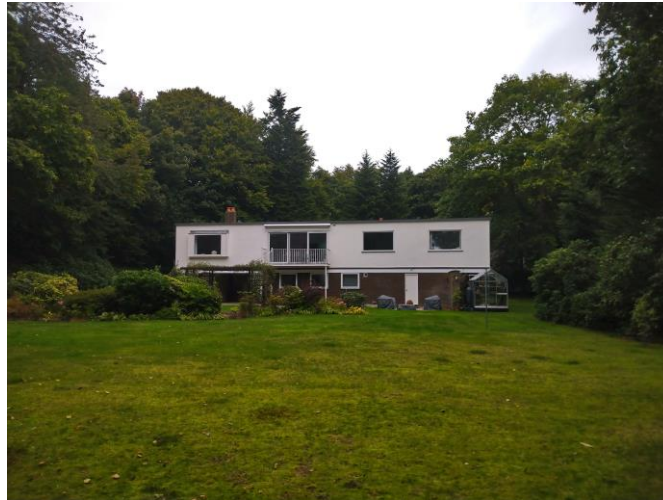
View of rear elevation
