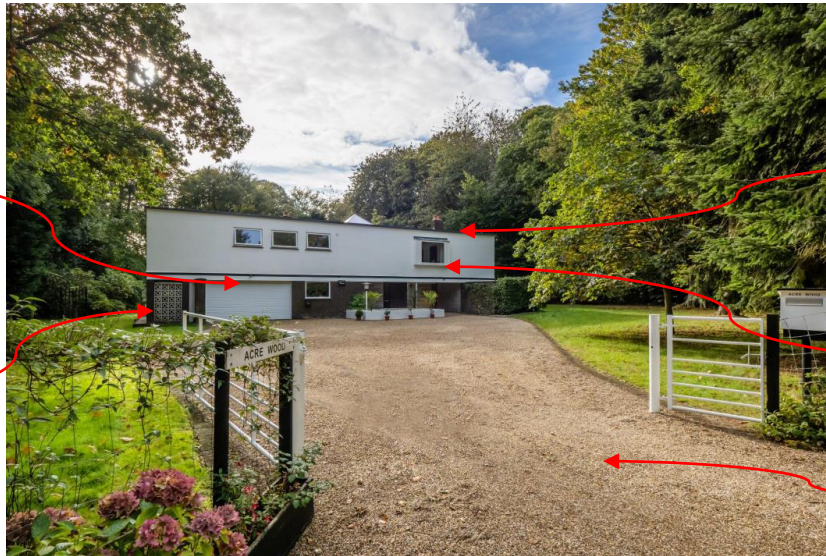
View of the existing building from the front
