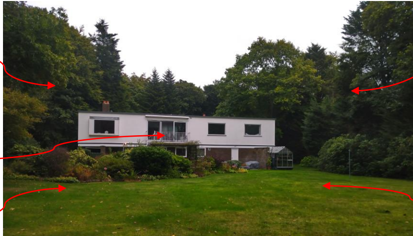
View of the existing building from the rear
