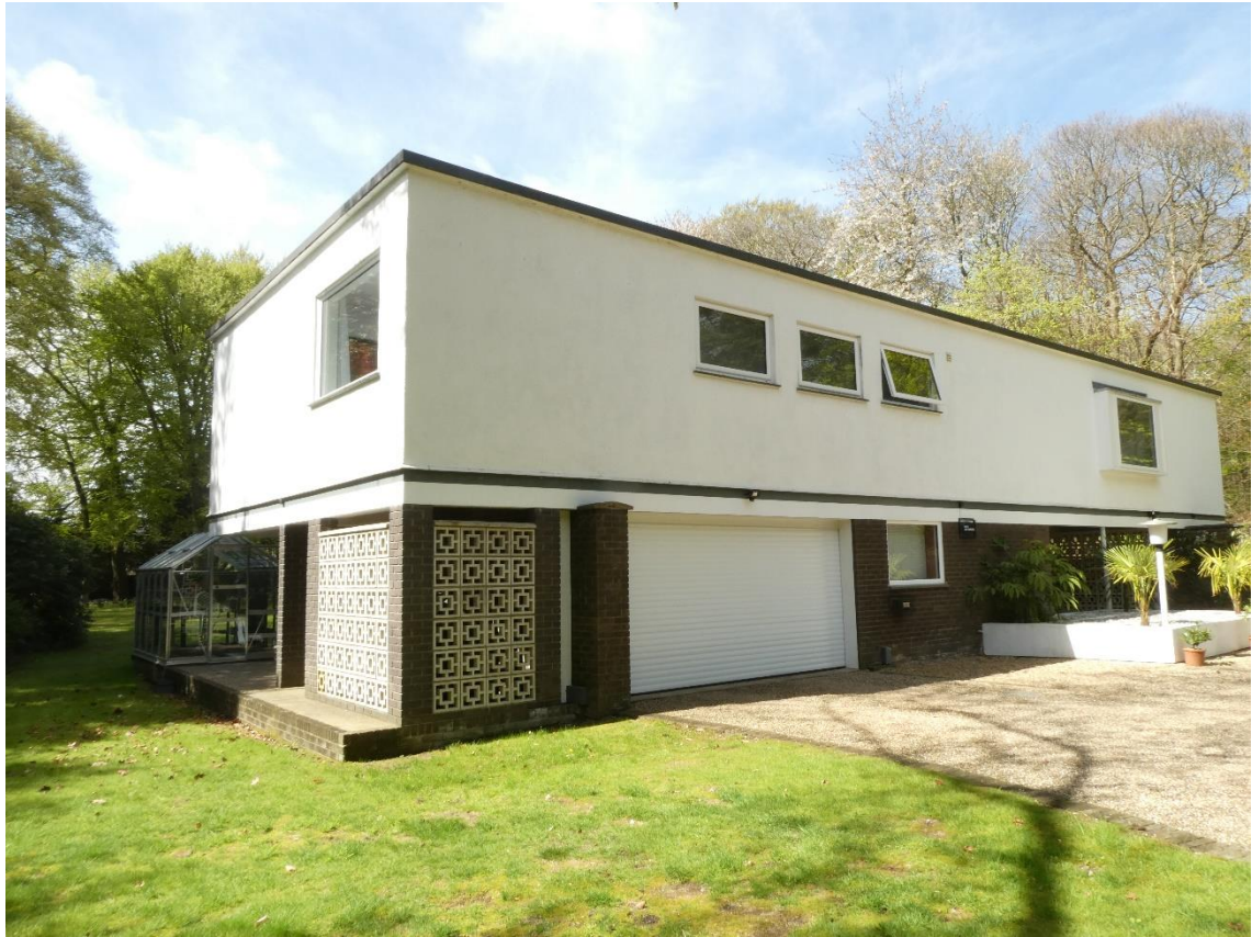
Photo 1 , north and east aspects of building one, looking southwest.
