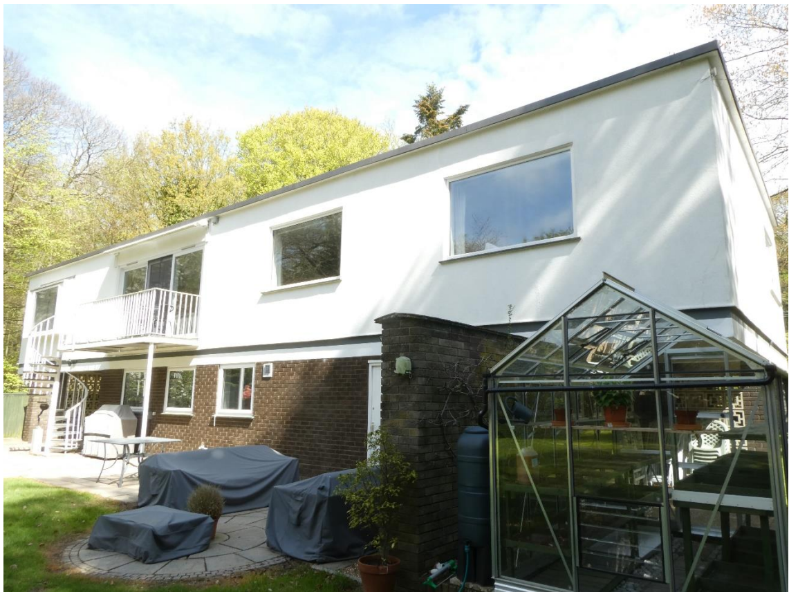
Photo 2 , south and east aspects of building one, looking northwest.
