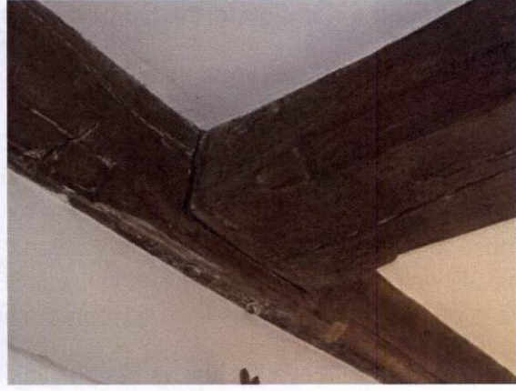
Left: ovolo moulded ceiling joist with lamb's tongue stop, supported by decorated bracket on principal post at NE corner of hall, looking into SE end of cross passage with secondary stair door opposite and rear door on right; Right: axial beam with ovolo moulding meeting joist on SW side of cross passage with plastered brick wall for reduction beneath
