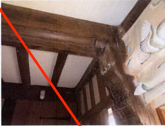
Left: ovolo moulded ceiling joist with lamb's tongue stop, supported by decorated bracket on principal post at NE corner of hall, looking into SE end of cross passage with secondary stair door opposite and rear door on right; Right: axial beam with ovolo moulding meeting joist on SW side of cross passage with plastered brick wall for reduction beneath
