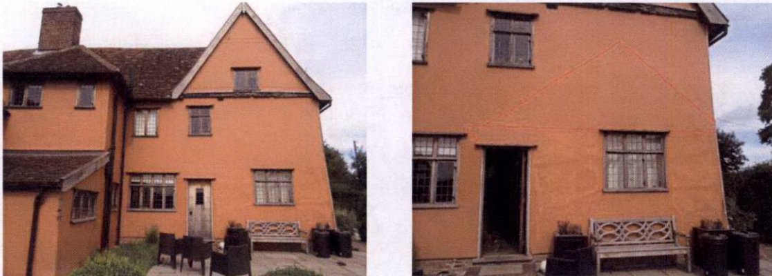
Left: SE (rear) elevation showing site of proposed extension; Right: imprint in render of roofline of 1960s extension (demolished in 2006) outlined in red on image
