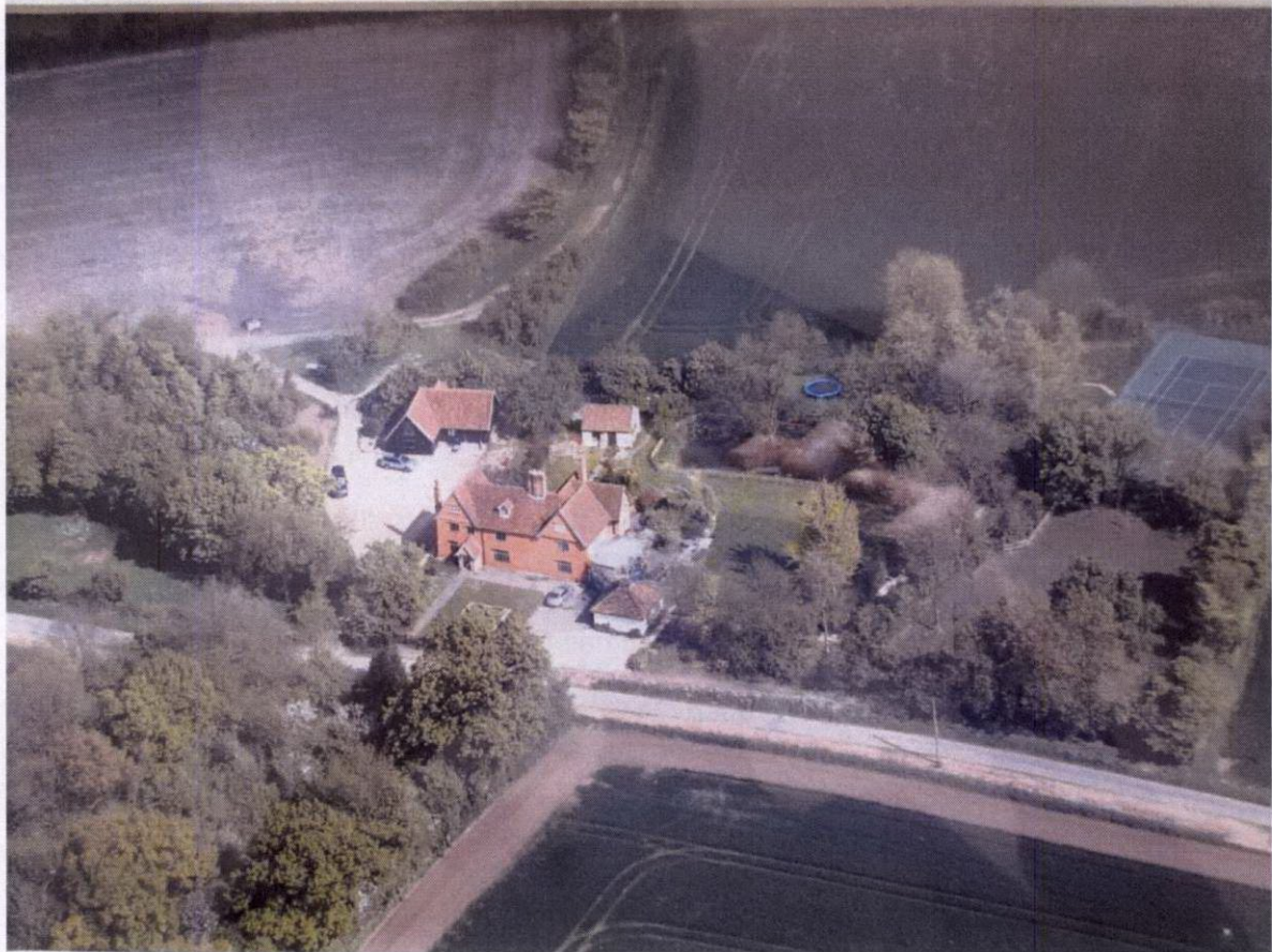
2005 Aerial photograph (by kind permission of Mr & Mrs Carrington) This shows Mollands Barn to the NE of the house, the garden shed (now demolished) to the SE, the garage, link wall and SW extension (all demolished)
