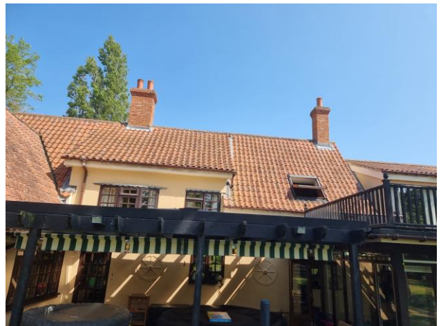
Photo 4: closer view of the roof on the south of the property.
