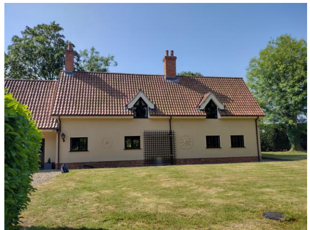
Photo 10: View of the north of the property of the main building.
