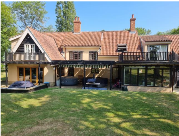
Photo 3: View from the south of the property where the proposed single storey extension will go.
