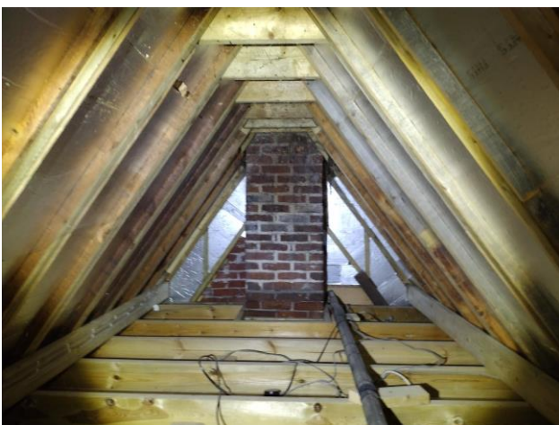
Photo 5: Internal attic of the main building.
