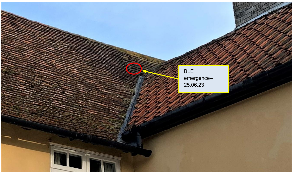
Plate 3.6: Emergence point on south-eastern slope of main roof – brown long-eared on 25/06/23.
