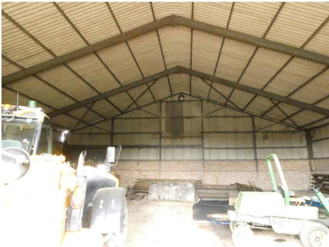
Photo 6 , internal view of building one, looking north.
