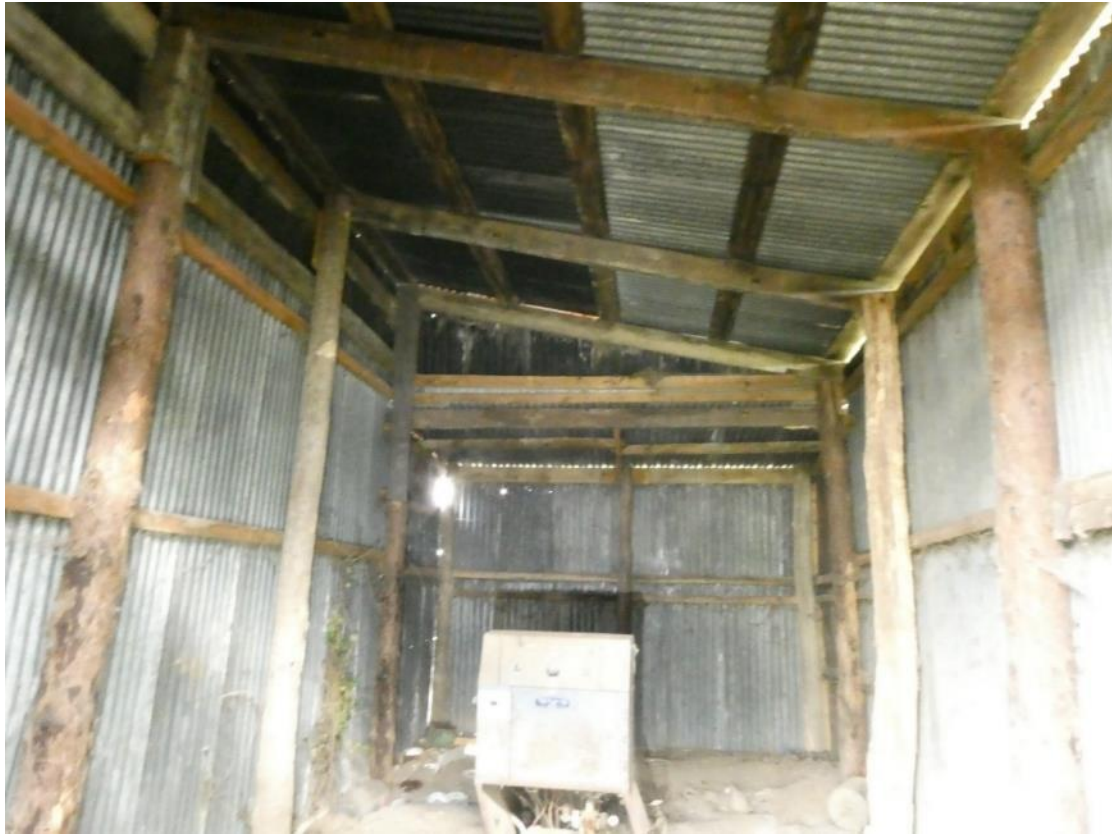
Photo 8 , internal view of building two, looking north.
