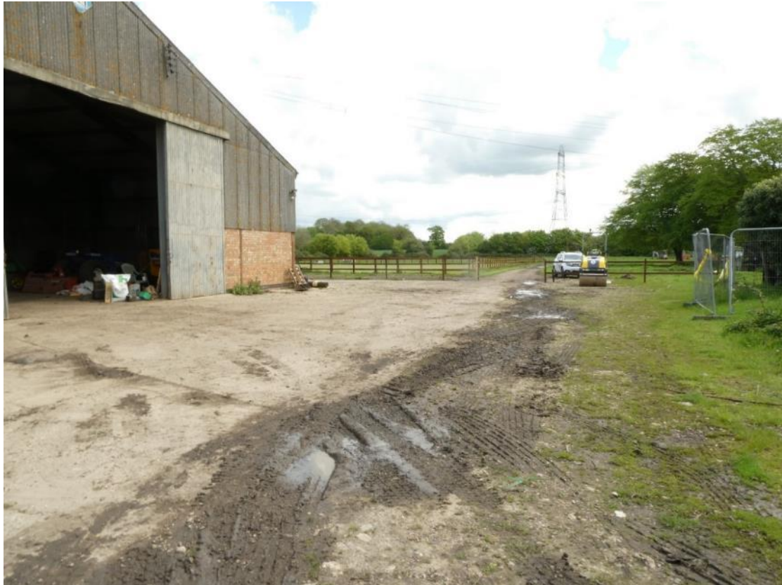
Photo 1 , area of concrete and compact gravel hardstanding to the southeast of the site, looking east.
