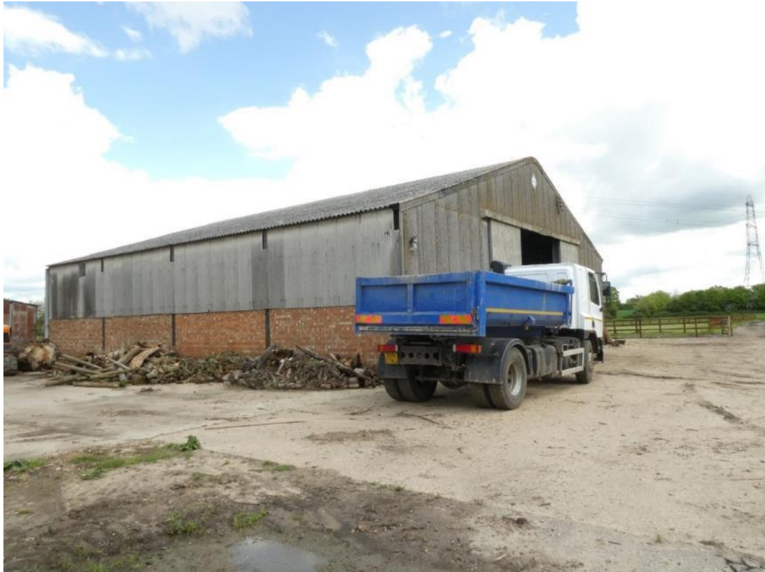
Photo 5 , south and west aspects of building one, looking northeast.
