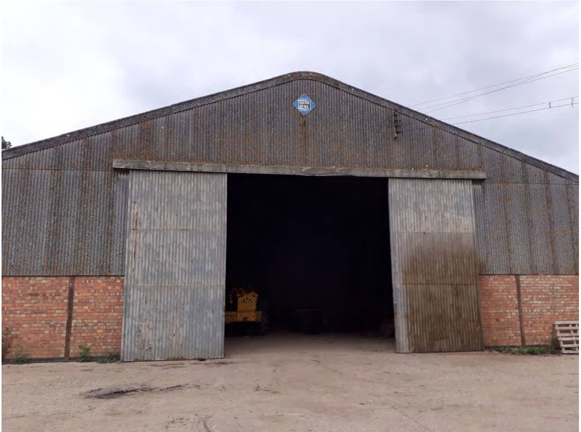
Photograph 1: Front elevation of barn (south side)
