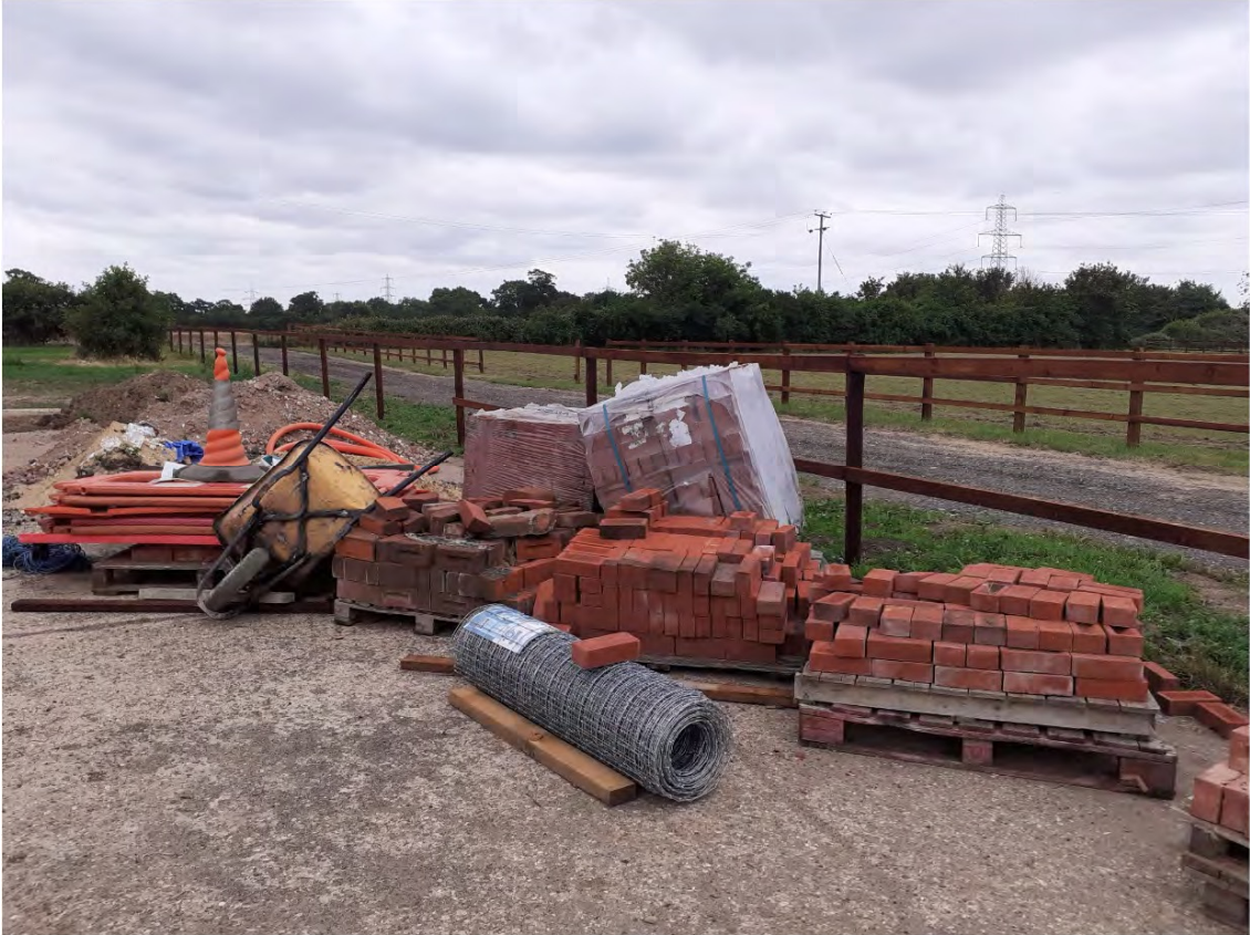
Photograph 5: Building materials stored on concrete east side
