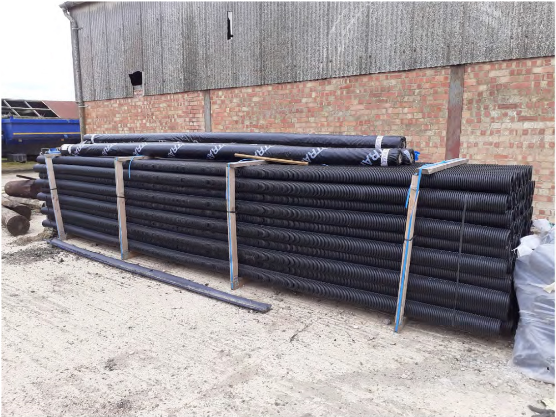
Photograph 7: Drainage pipes stored on slab
