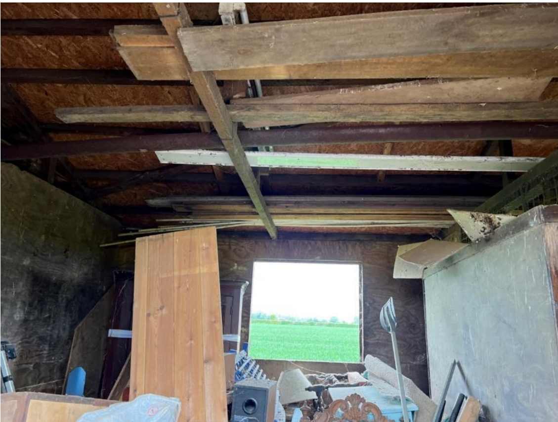
Photo 18. View of unit B1d, building 1.
