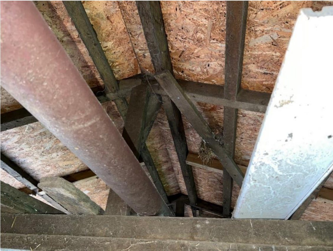
Photo 52. Swallow nest within rafters of the stables, building 1. Unit B1d.
