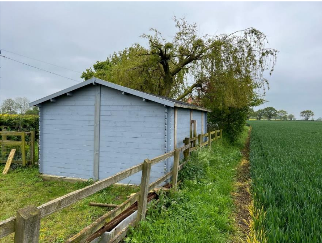
Photo 22. View of building 3 and willow (T2)
