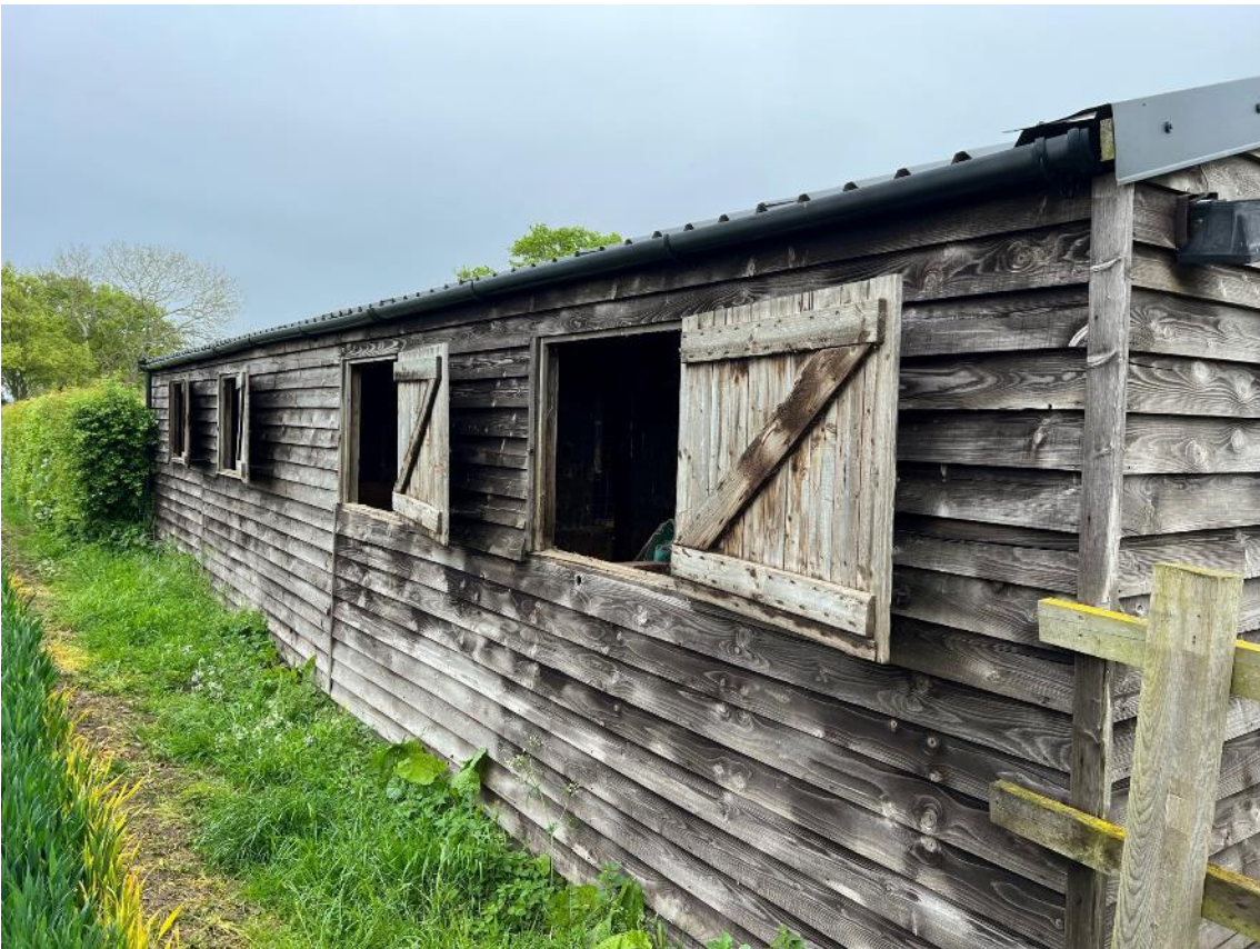
Photo 5. Rear of the stables, building 1.
