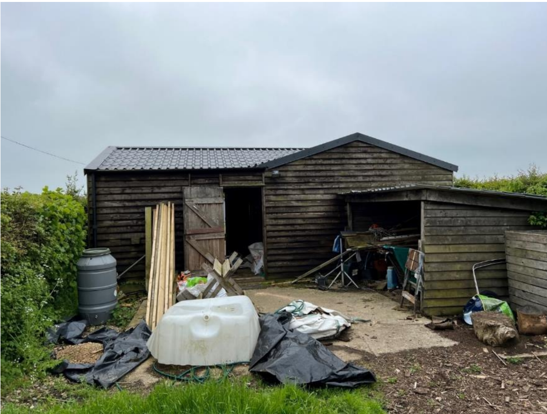
Photo 21. View of building 1 and building 2. Shows concrete pad.
