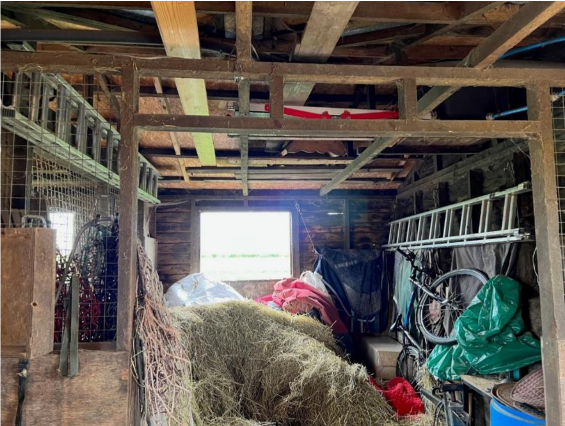
Photo 11. View of unit B1a, building 1.
