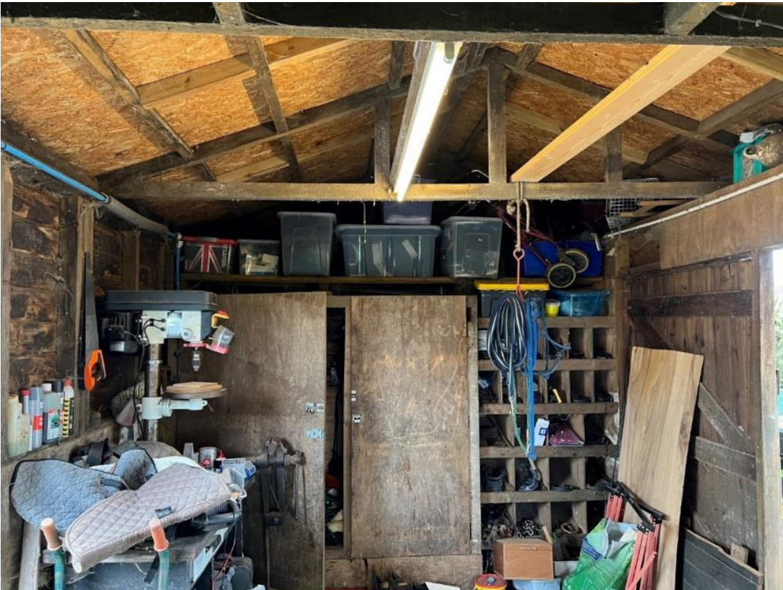
Photo 12. View of unit B1a, building 1.
