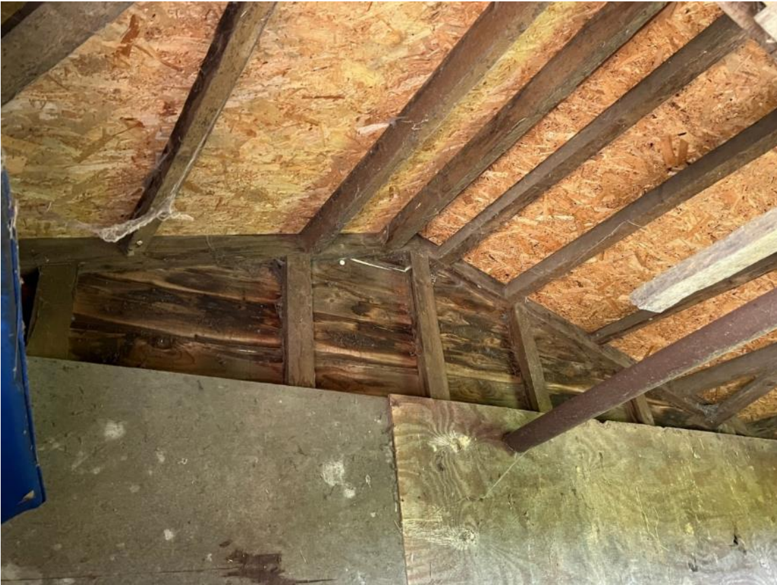
Photo 19. View of unit B1d, building 1.
