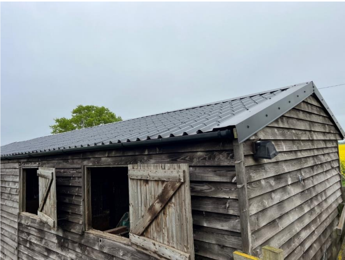
Photo 6. Rear of the stables, building 1.
