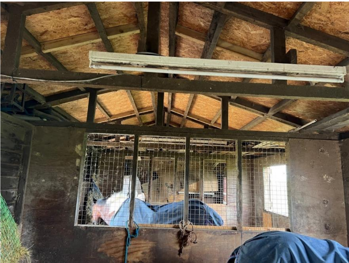
Photo 14. View of unit B1b and B1c, building 1.
