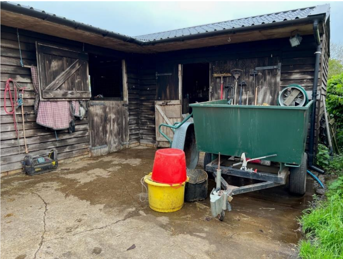
Photo 2. The stables, building 1. View from concrete pad/driveway. Looking at unit B1a and B1b (left to right).
