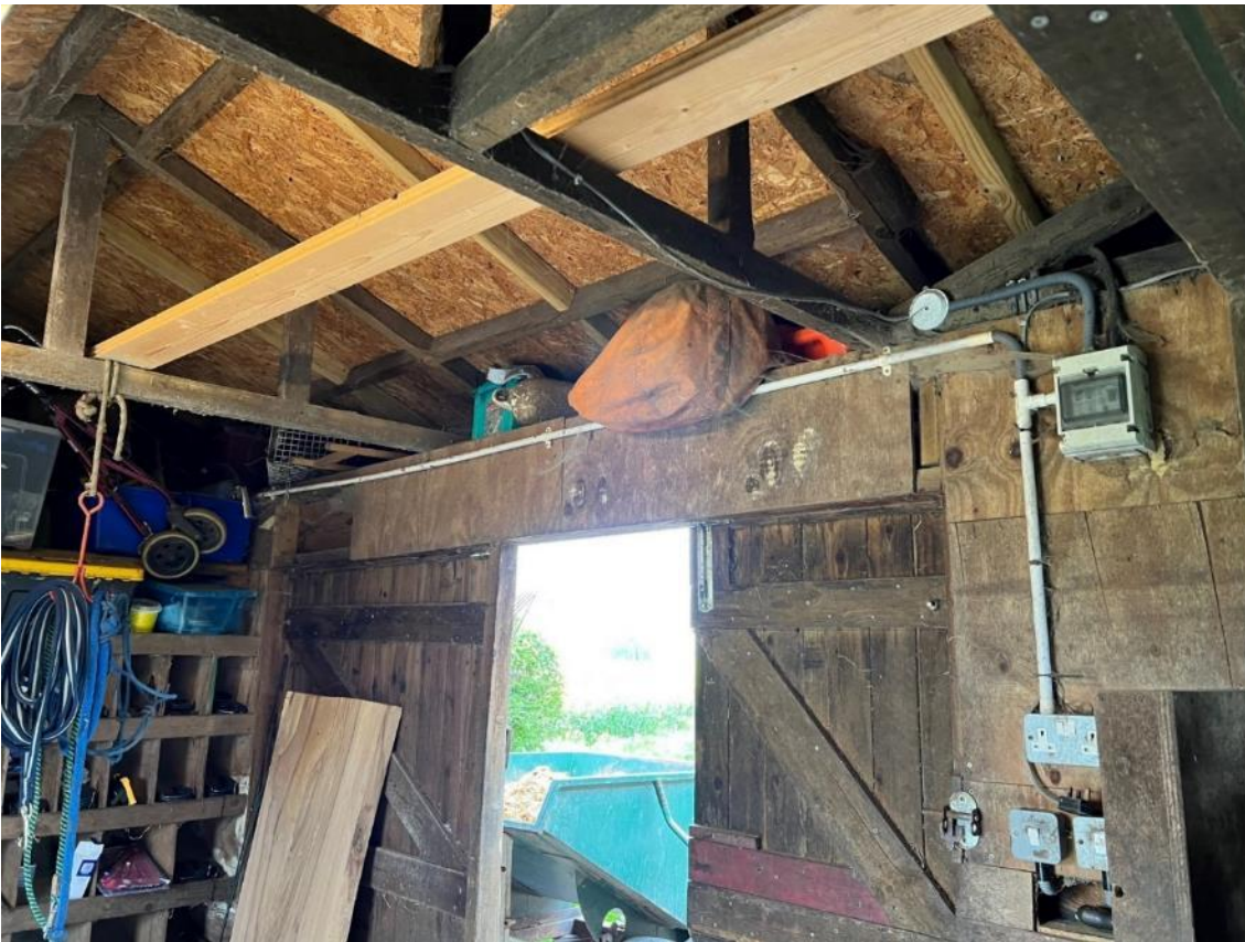
Photo 13. View of unit B1a, building 1.
