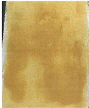
Limewash during drying
