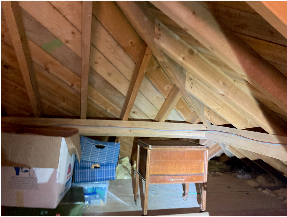
Photograph 3: Internal view of roof space.
