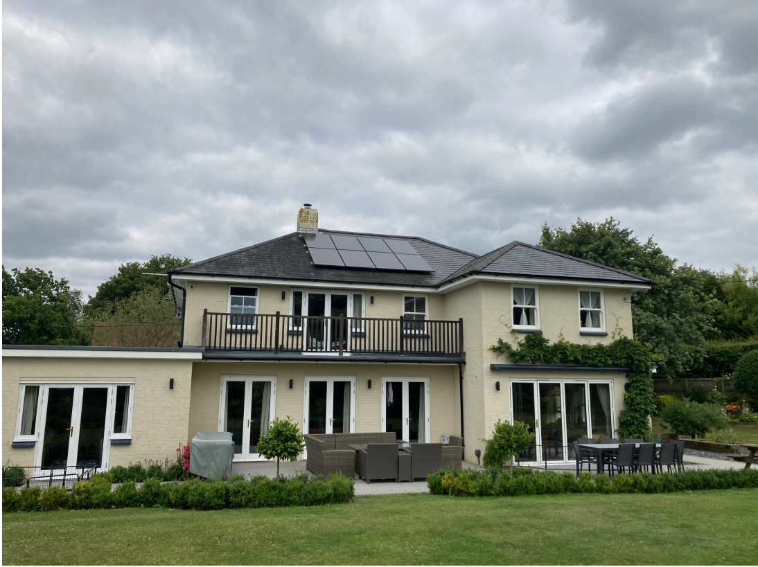
Photograph 1: Eastern side of building.
