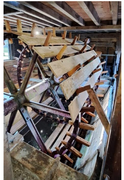
Re assembly of Whitchurch Silk Mills Waterwheel
