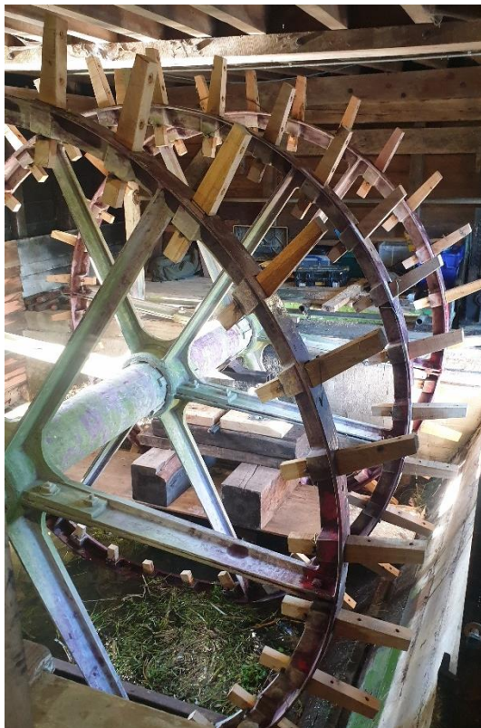
Re assembly of Whitchurch Silk Mills Waterwheel
