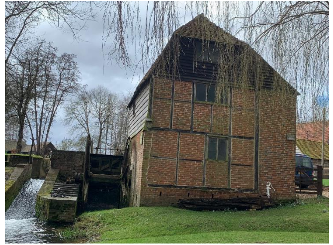
View of the Mill, Downstream from the North
