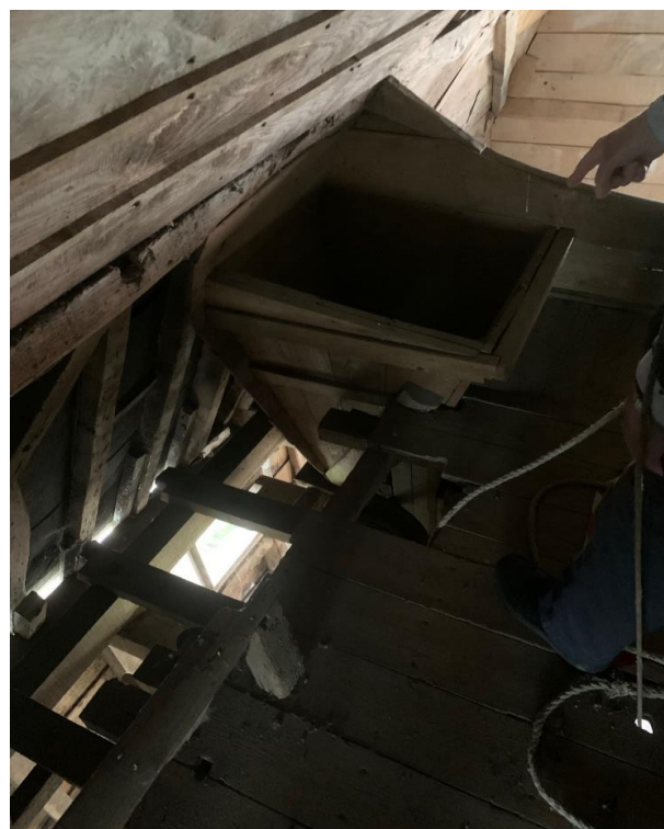
The Hoist pulleys and mechanism seen here with the owner of the Mill will be retained as part of the refurbishment plans. However, the upper floor of the bin floor will be removed together with some of the grain bins to facilitate the new layout. Hoppers will be retained where possible and an illustrative graphic with technical description of the bin floor mounted nearby on the wall.
