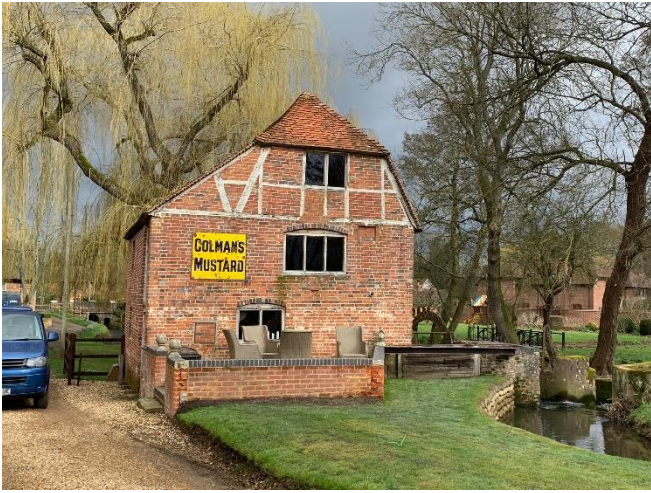
View of the Mill, Upstream from the South
