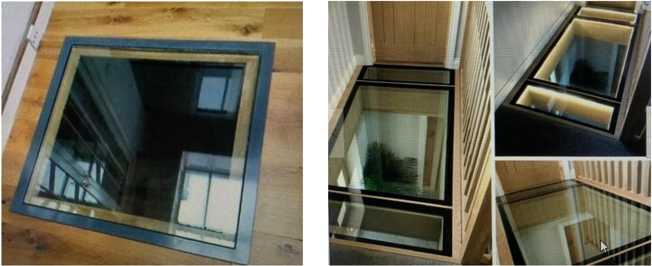
Examples of toughened and laminated structural glass flooring
