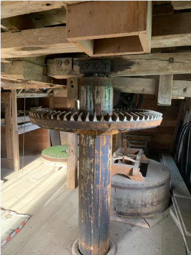
The Stone Floor (First floor) – The Hopper, Crown wheel and Mainshaft will be retained as part of the refurbishment plan. These elements will be cleaned, repaired as necessary and painted in dark grey. Note the sack flaps, bottom left of this photo to be retained.
