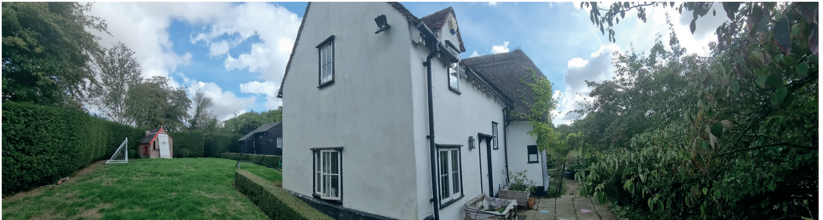
07 View of Rear Elevation
