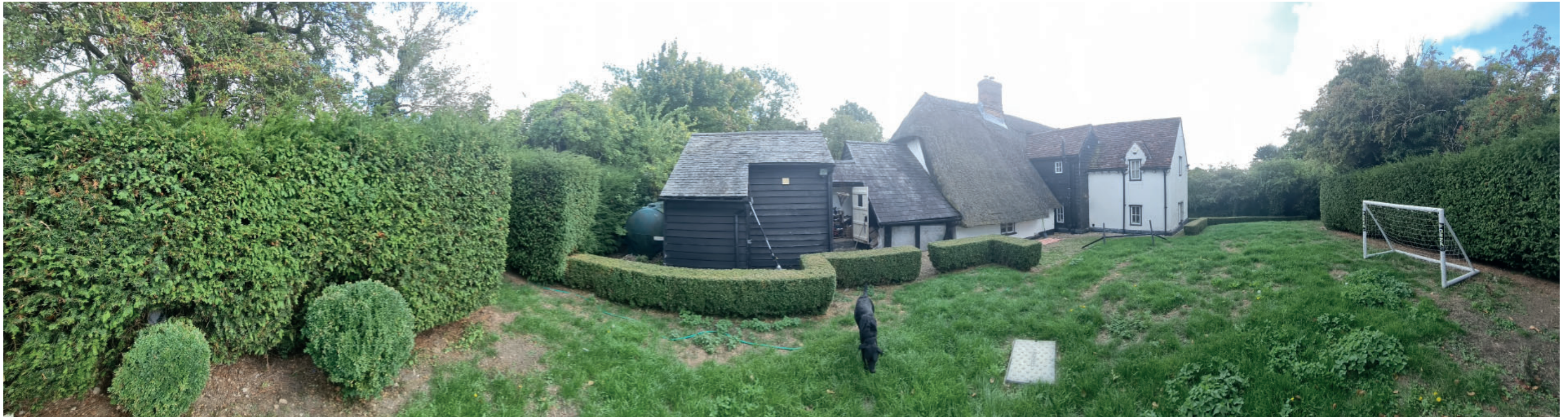
04 View of Rear Elevation
