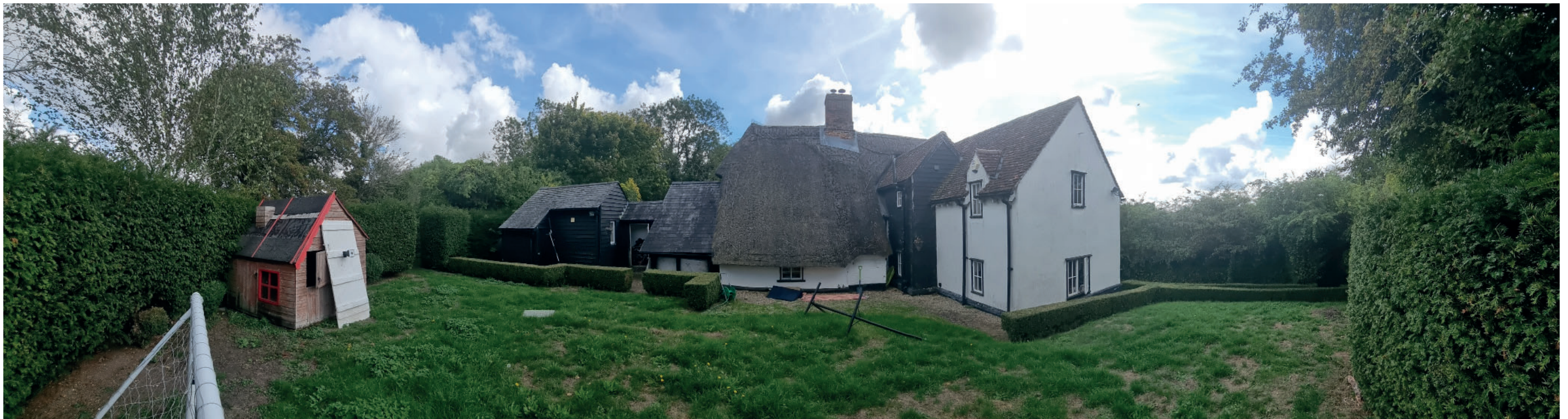
05 View of Rear Elevation
