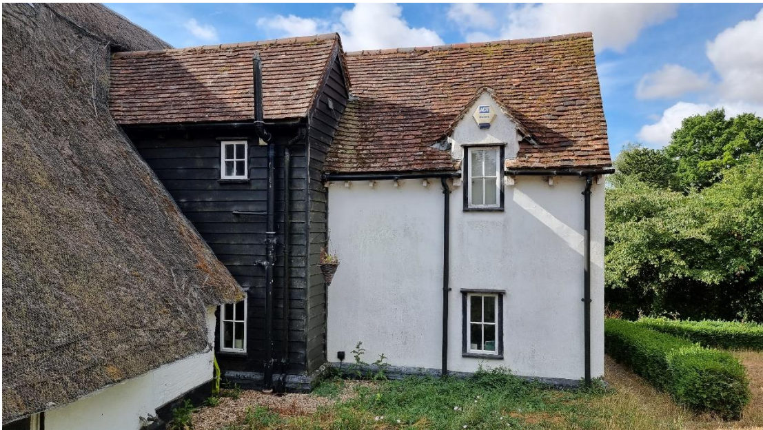
Fig.5: The north elevation of the rear addition.
