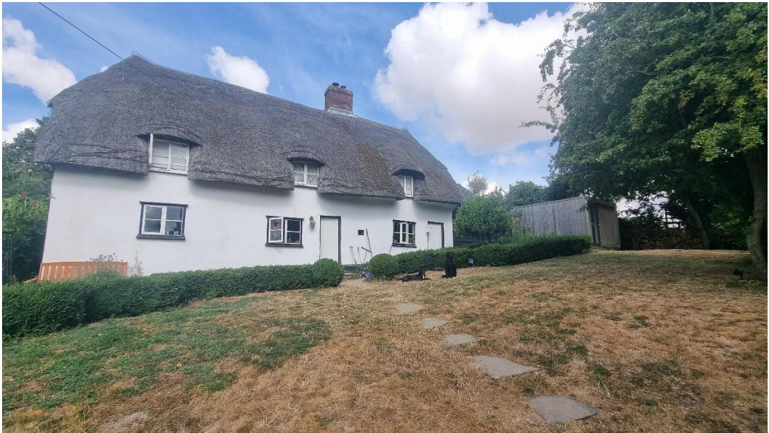
Fig.2: The east elevation of the property is the oldest part of the property and is of timber frame construction, finished in white render. The thatch roof is a style once common in Brent Pelham, however many other properties in the village were reroofed with slate or tile in the 20 th century. The single storey timber clad structure seen to the right of the house is a detached studio.
