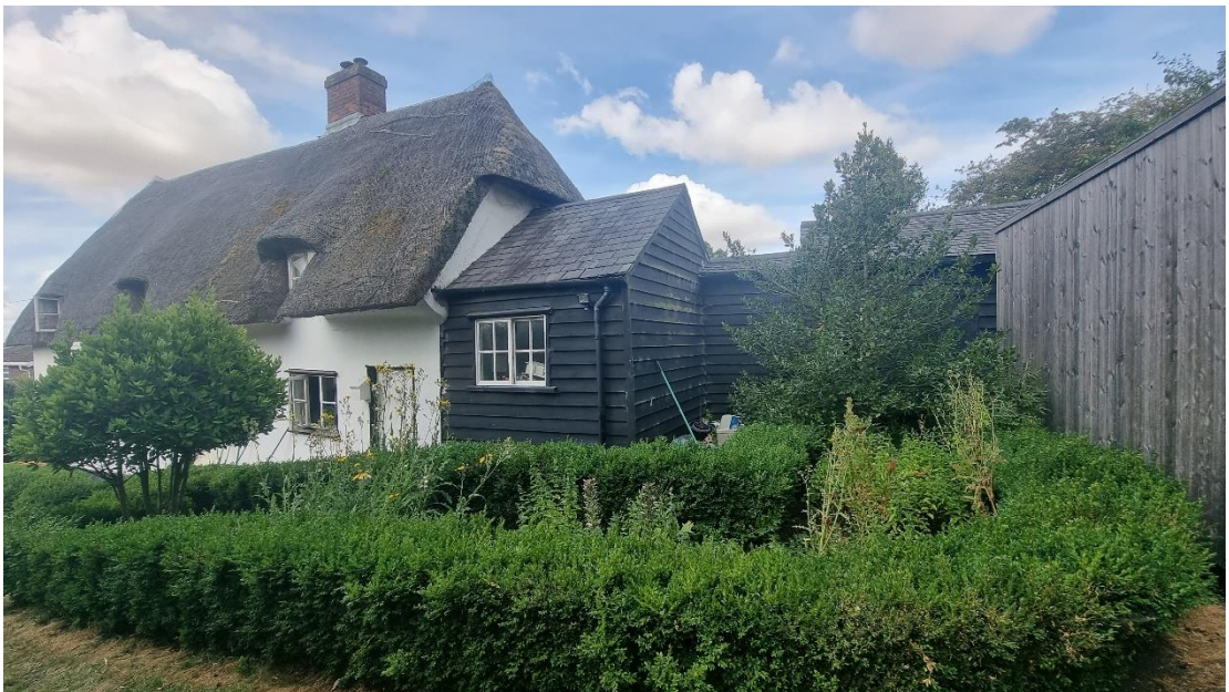
Fig.3: The post construction additions to the north elevation are clad in weatherboard with slate roofs, the modern detached studio can be seen to the right of the image.
