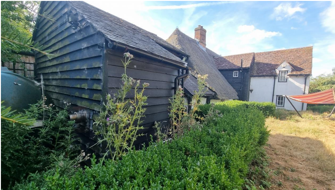
Fig.6: The weatherboarded single storey additions to the north elevation are traditional in style but are late 20 th century.
