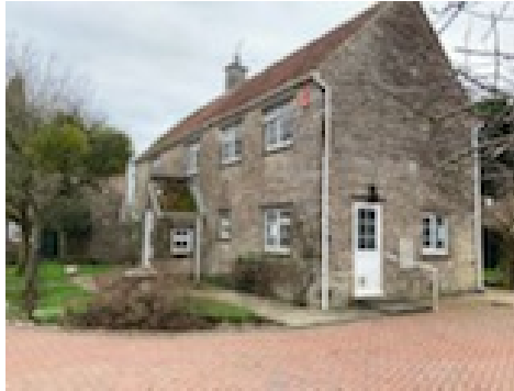
Existing northeast facade
