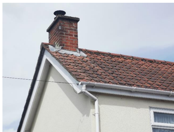
No gaps under tile or around chimney or under lead flashing.
