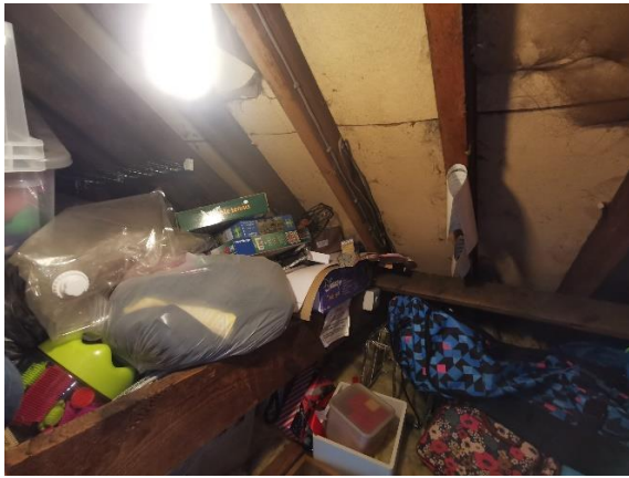
Exposed beams and boarding.
