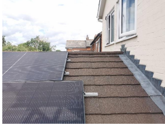
Sealed roofing with no gaps to the rear of the Site.
