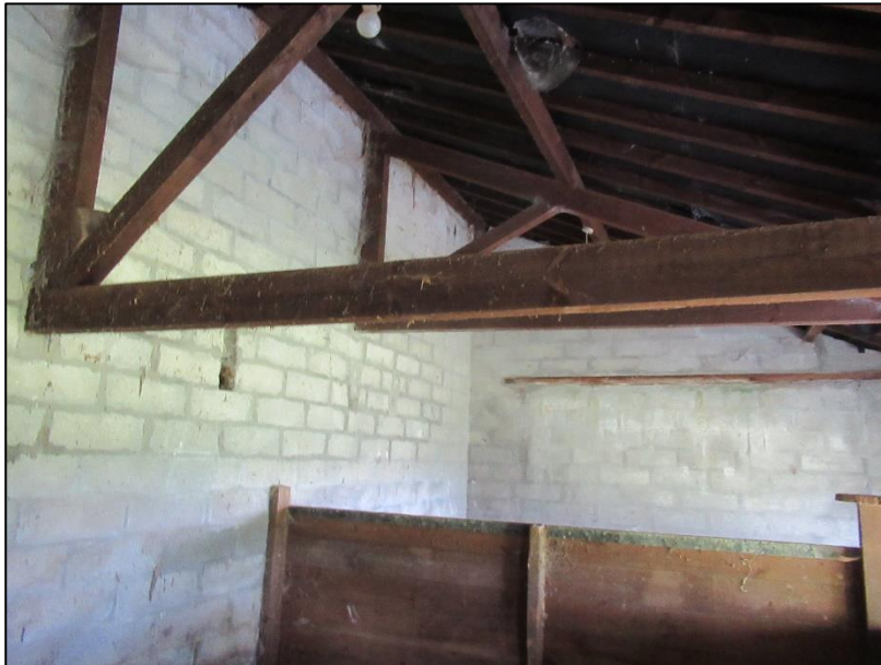
Monopitch trusses within the modern west barn supporting the roof structure.
