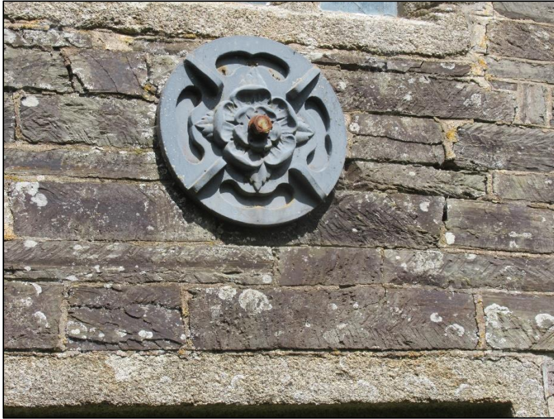
Pattress plate set between the eastern windows within the front elevation.
