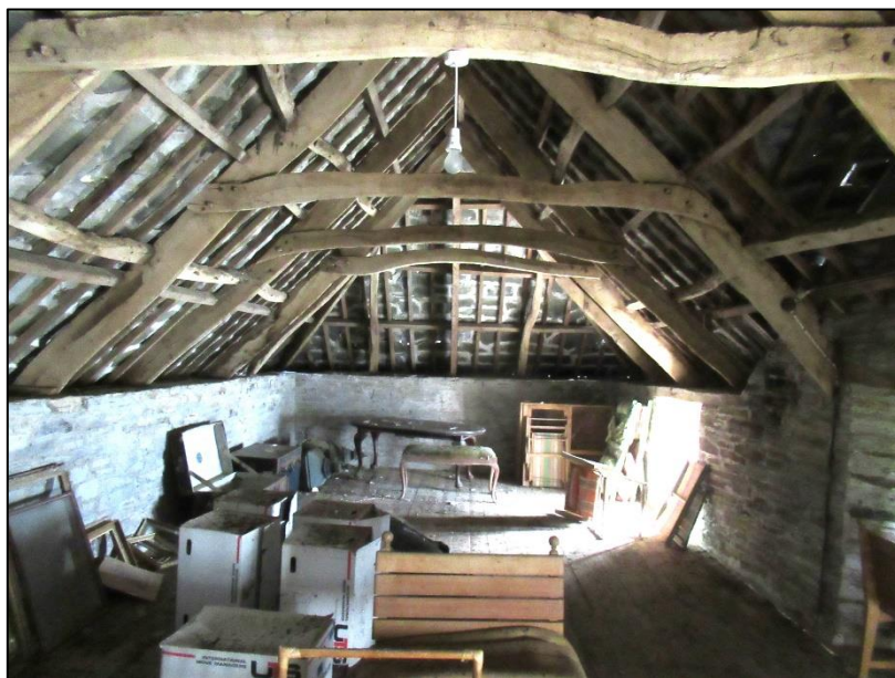
Original primary A frame oak trusses with later purlins & common rafters.
