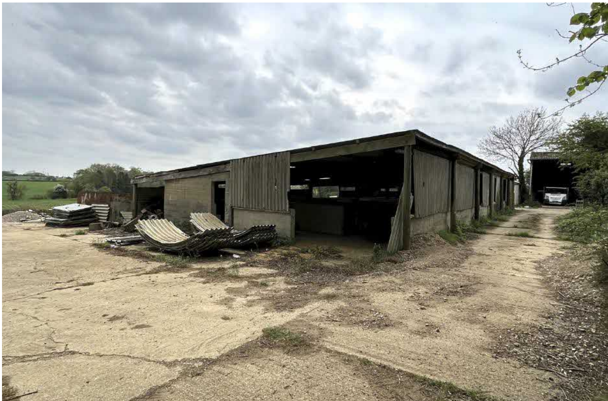
Photo 5. B1 north side, showing surrounding hardstanding
