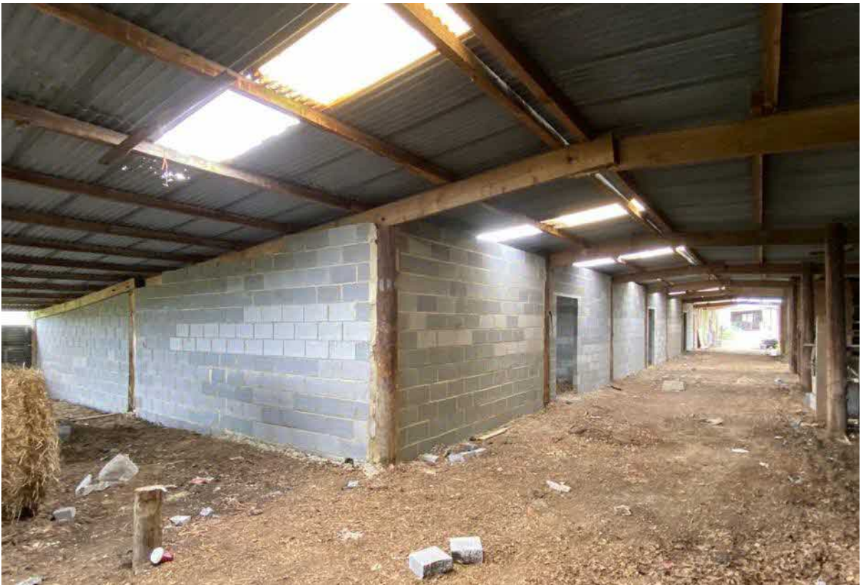
Photo 9. Interior of B3
