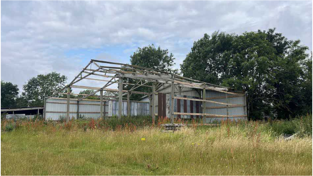
Photo 7. Barn 2 (B2) taken from the southeast corner looking northwest
