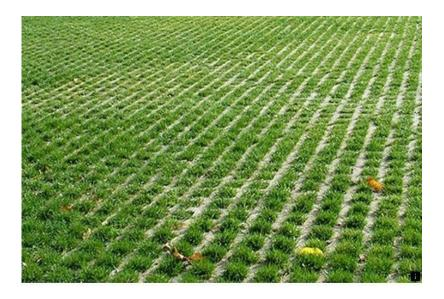
As can be seen this is essentially a Grass paving, requiring no excavation and can be installed over existing grass allowing grass to grow through the cell's providing a natural grass surface suitable for the use of the vehicles. It is a commonly used product and one which will benefit and improve the area in question and minimises the impact on the Green Belt.
