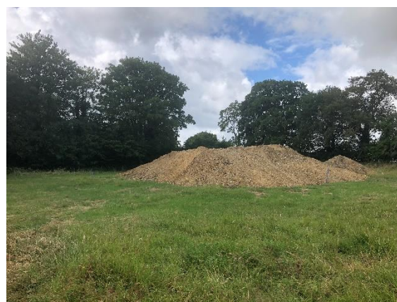
View of entire works area.
