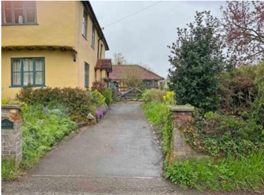
Fig.13 View in Groton Road with the vehicular access aligned on the 1997 annex to the rear of the curtilage to Cotelee and the site of the link obscured by the listed building
