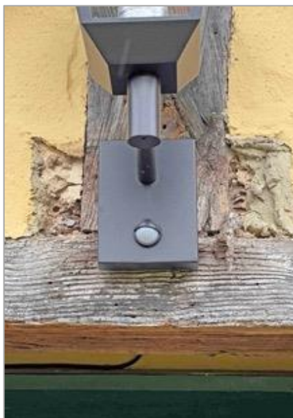
Fig.8 Use of hard cement render & metal lath
