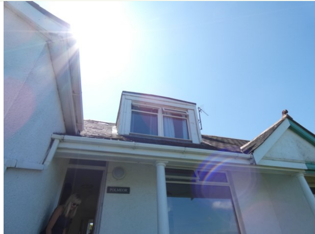
North-west elevation: Bargeboard, fascia and soffits all tight fitting and in good repair. Slates and leadwork around dormer tightfitting.
