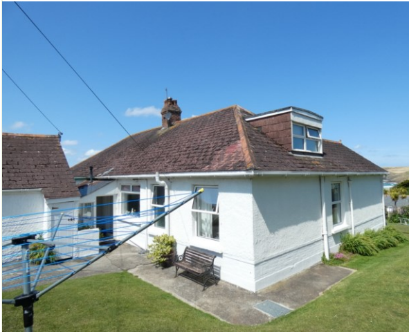
Polmeor, southeast elevation: Slates appear tight and secure with no gapping.
