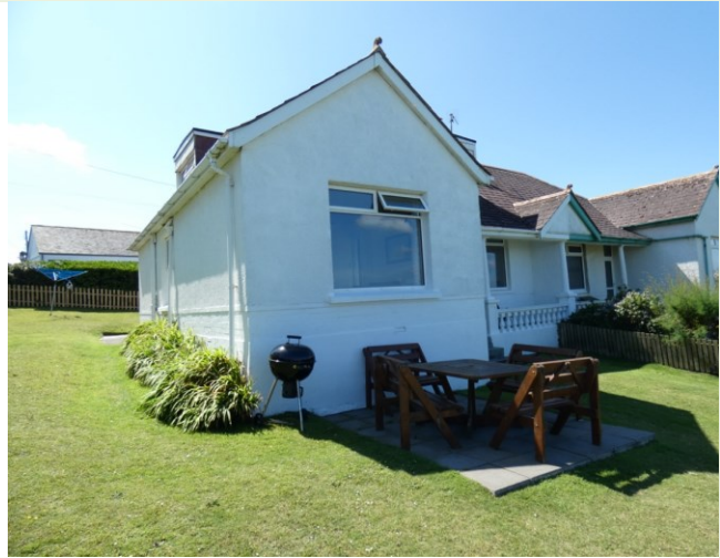
Northern Elevation: Bargeboard and soffits in good repair and tight fitting.
