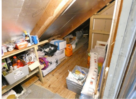
Vaulted Ceiling: Unlined and insulated with fiberboard.
