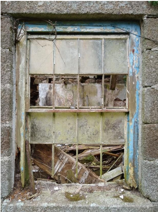
Figure 9. 16 pane sash windows on west elevation
