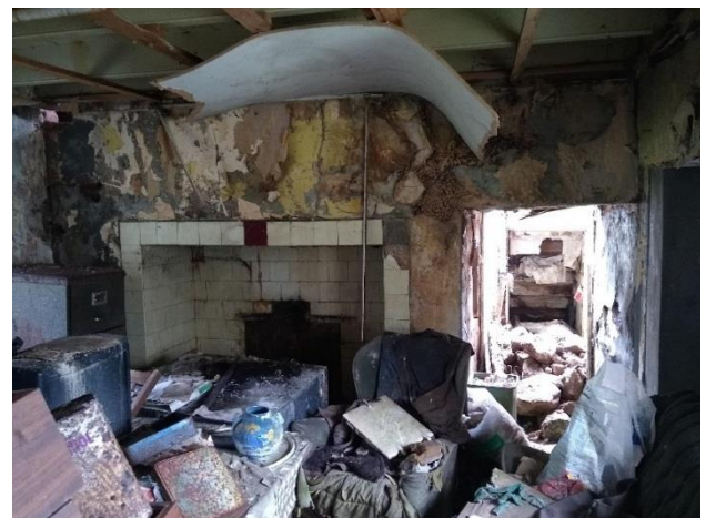
Figure 12. C17 living room, showing main hearth and passage to C19 house
