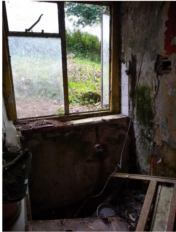
Figure 6 Cement render inside the infilled door opening on the southern elevation
