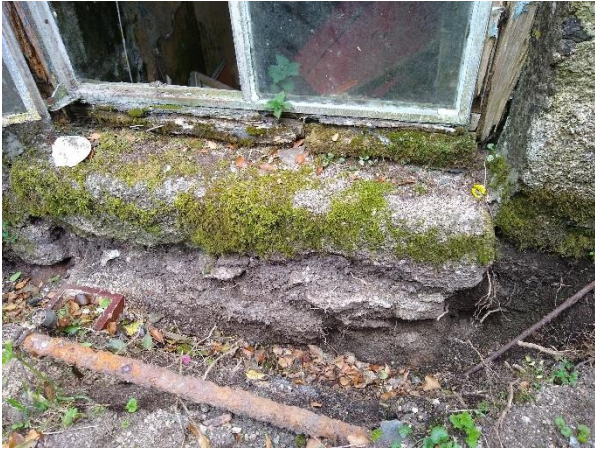
Figure 5 Infilled stonework and reused lintel below window on southern elevation
