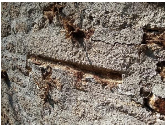
Figure 20 Chamfered lintels inbuilt into walls of farmhouse
