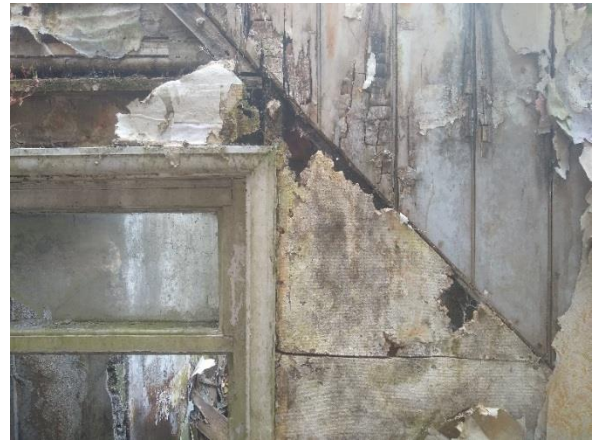
Figure 16 Boarded partition partitioning stairs in left hand room
