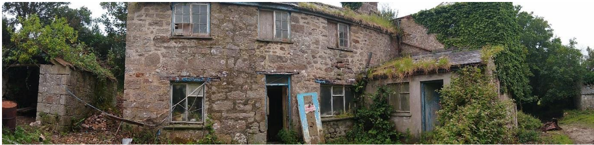
Figure 3 Showing the northern elevation of the C17 farmhouse
