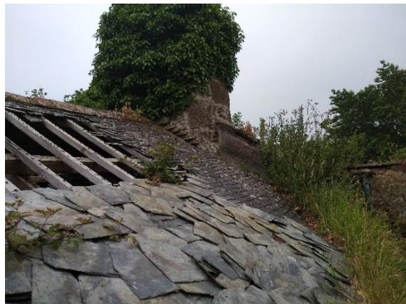
Figure 10 Scantle roof and main stack
