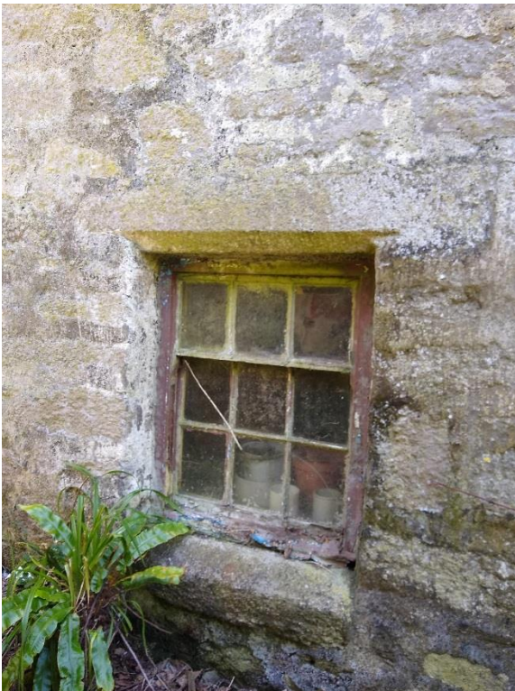
Figure 7 Window on eastern elevation and bag rubbed granite rubble walls
