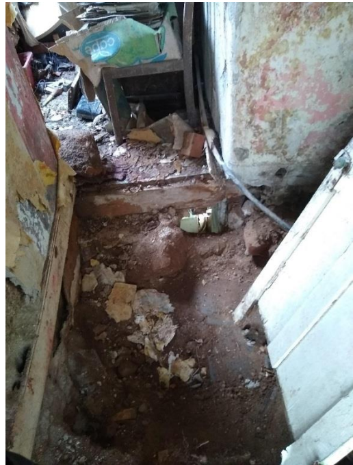
Figure 14. Slate floor tiles around old stairwell in C17 house
