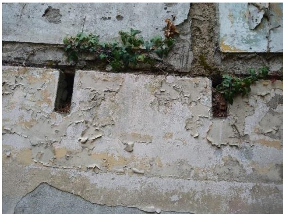
Figure 17 Evidence of exposed beams in left hand groundfloor room of C19 house.
