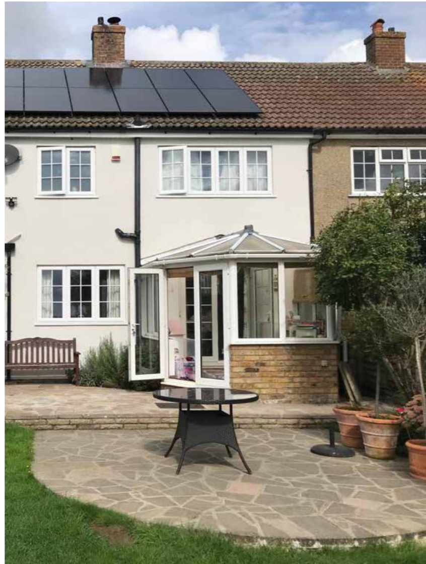
view showing the existing conservatory (to be removed)
