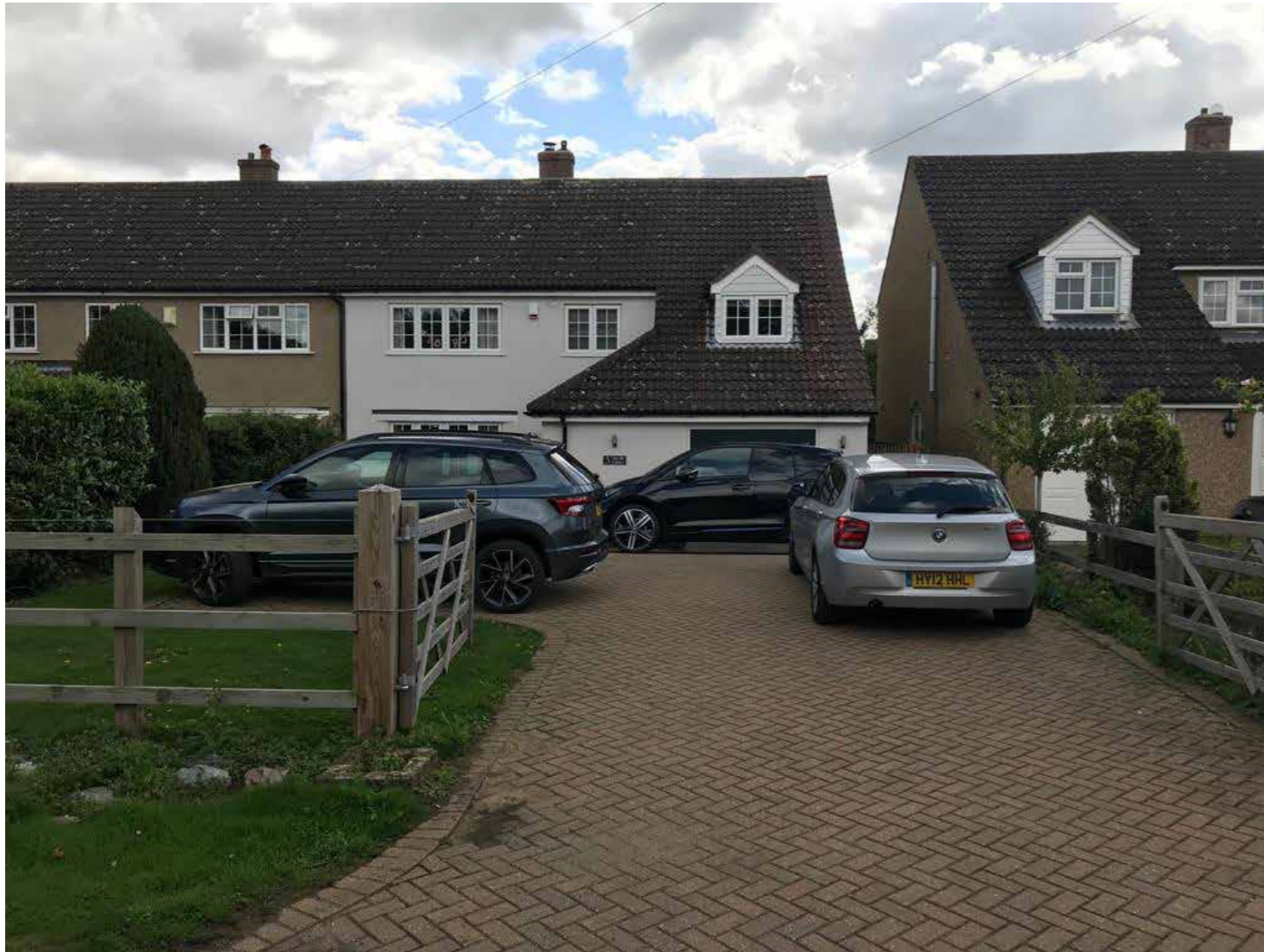
View showing the front elevation
