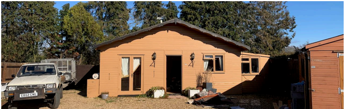
Photograph 1. Bungalow – south aspect
