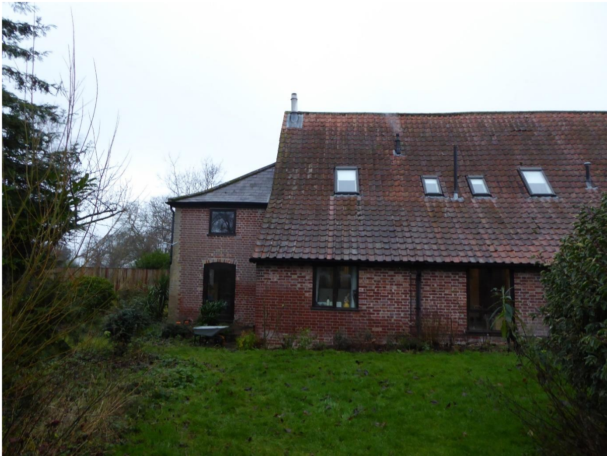
Photo of rear elevation of Lodge Barn South (2020).
