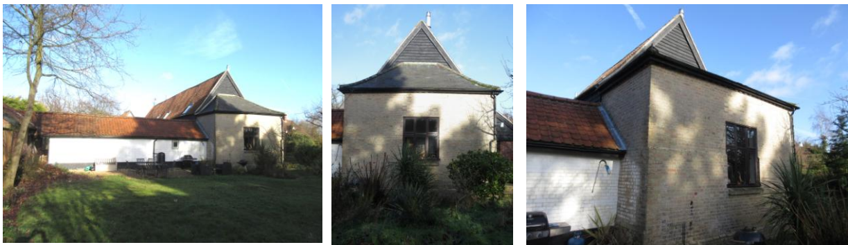
Left: looking N showing S elevation; Centre & Right: detail of white brick early 19th century hipped roof extension to S elevation of barn.
