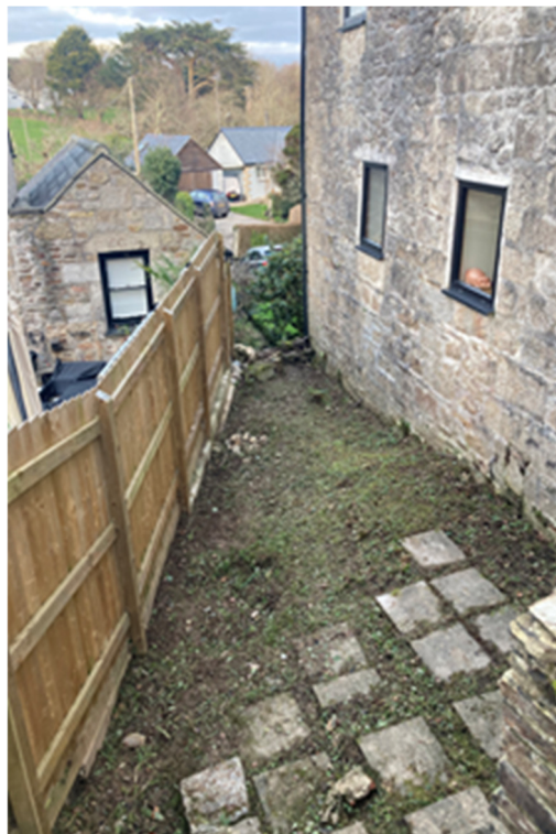
Figure 1: Rear yard tapering to northern end where there is a drop.
