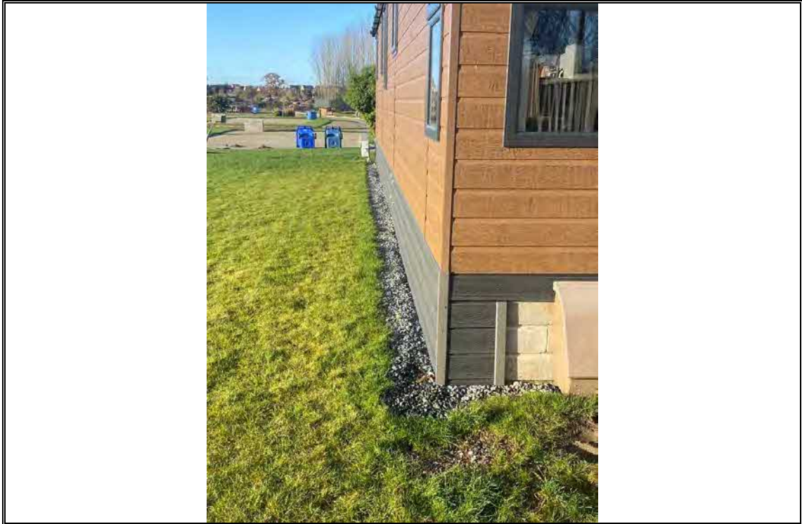
Photo OE/1702/1048 R1 PF2 – P05 –0.3m wide, 0.2 deep – gravel drainage at side of footpath and static caravan
