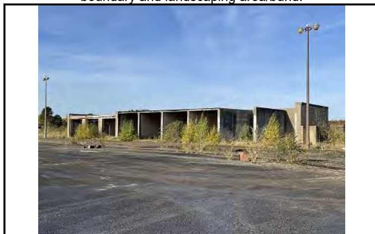
Photo OE/1702/1048/R1/P21 – Existing buildings on the site – to be refurbished.
