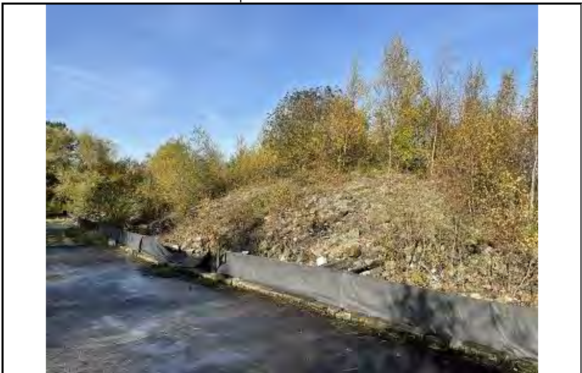
Photo OE/1702/1048/R1/P47 – Existing mound of crushed demolition waste – sampled and tested – see RSK Phase II Report 2021 – southern area of main site.
