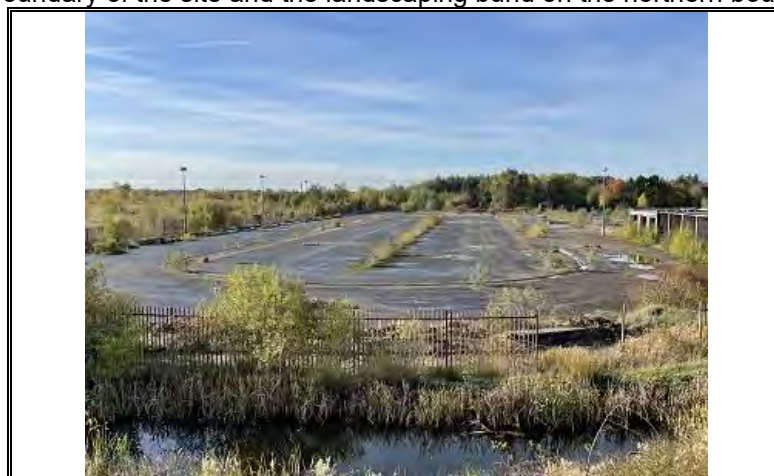
Photo OE/1702/1048/R1/P24 – View of pond and site from northern bund.
