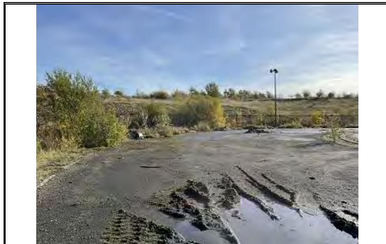
Photo OE/1702/1048/R1/P29 – View of northern boundary bund.
