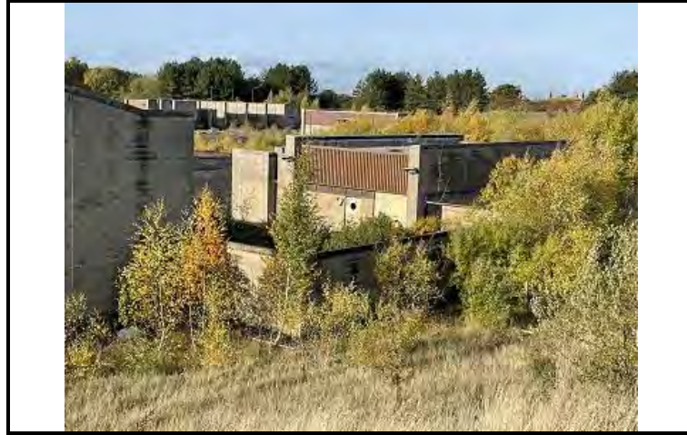
Photo OE/1702/1048/R1/P28 – Landscaped area and bunds on western side of the site.
