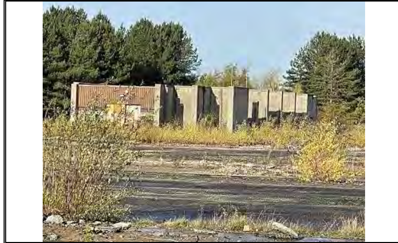
Photo OE/1702/1048/R1/P16 – Former buildings – looking southwest – to be refurbished.
