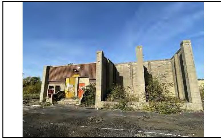
Photo OE/1702/1048/R1/40 – Existing buildings on the site – main electrical sub-station on the site – near western boundary.
