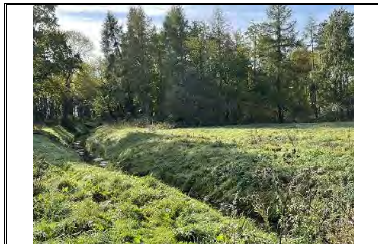
Photo OE/1702/1048/R1/P02 – View of drainage ditch on right hand side of site entrance
