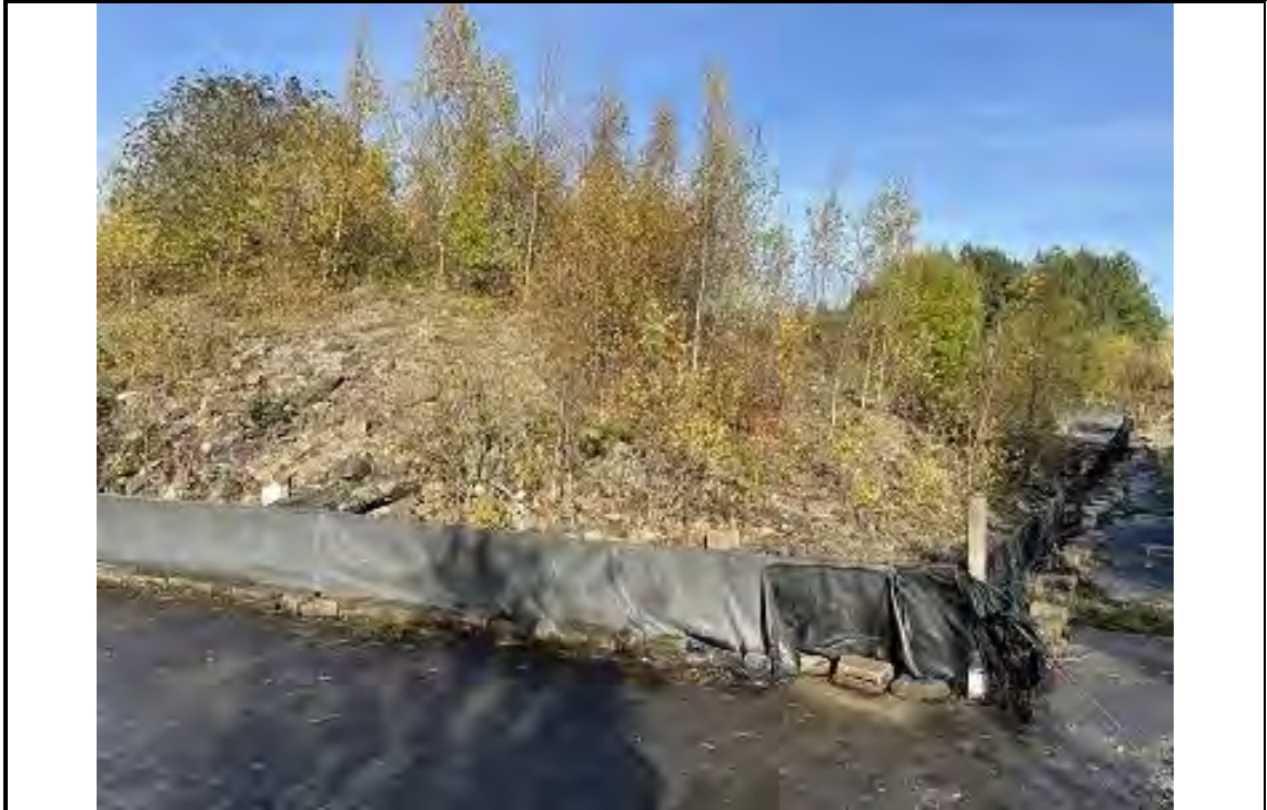
Photo OE/1702/1048/R1/P46 – Existing mound of crushed demolition waste – sampled and tested – see RSK Phase II Report 2021 – southern area of main site.
