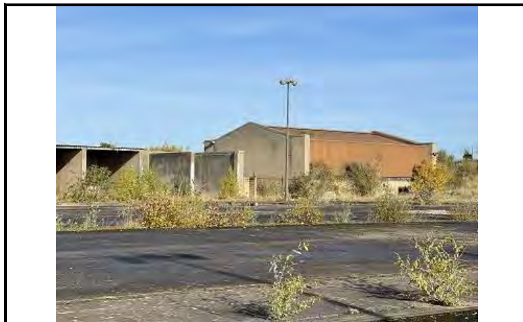
Photo OE/1702/1048/R1/P15 – Former buildings – looking southwest – to be refurbished.
