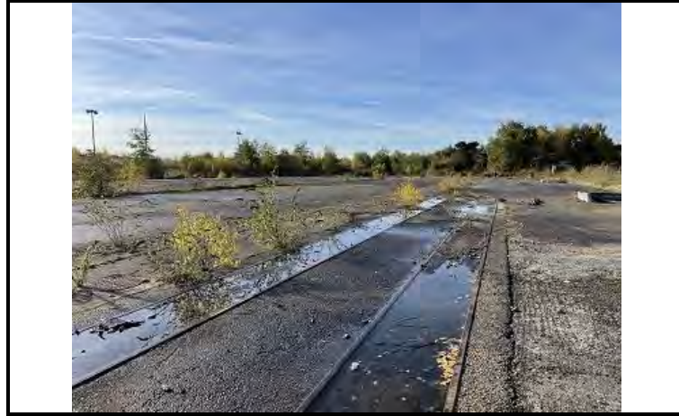
Photo OE/1702/1048/R1/P13 – View of mineral railway line within concrete slabs.
