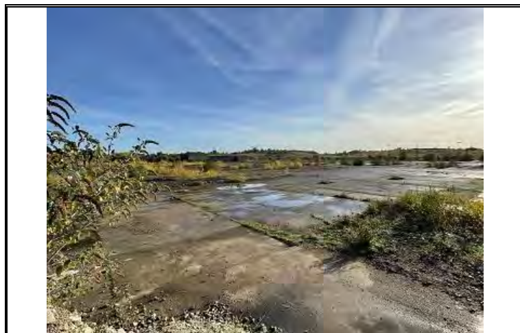
Photo OE/1702/1048/R1/P09 – General view of site and exposed concrete slabs – looking north.
