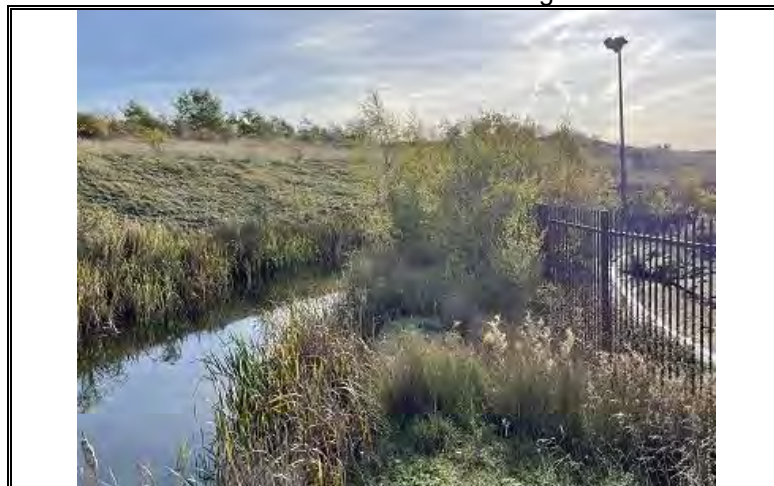
Photo OE/1702/1048/R1/P23 – Downstream collection pond from the storm water channels between the boundary of the site and the landscaping bund on the northern boundary.
