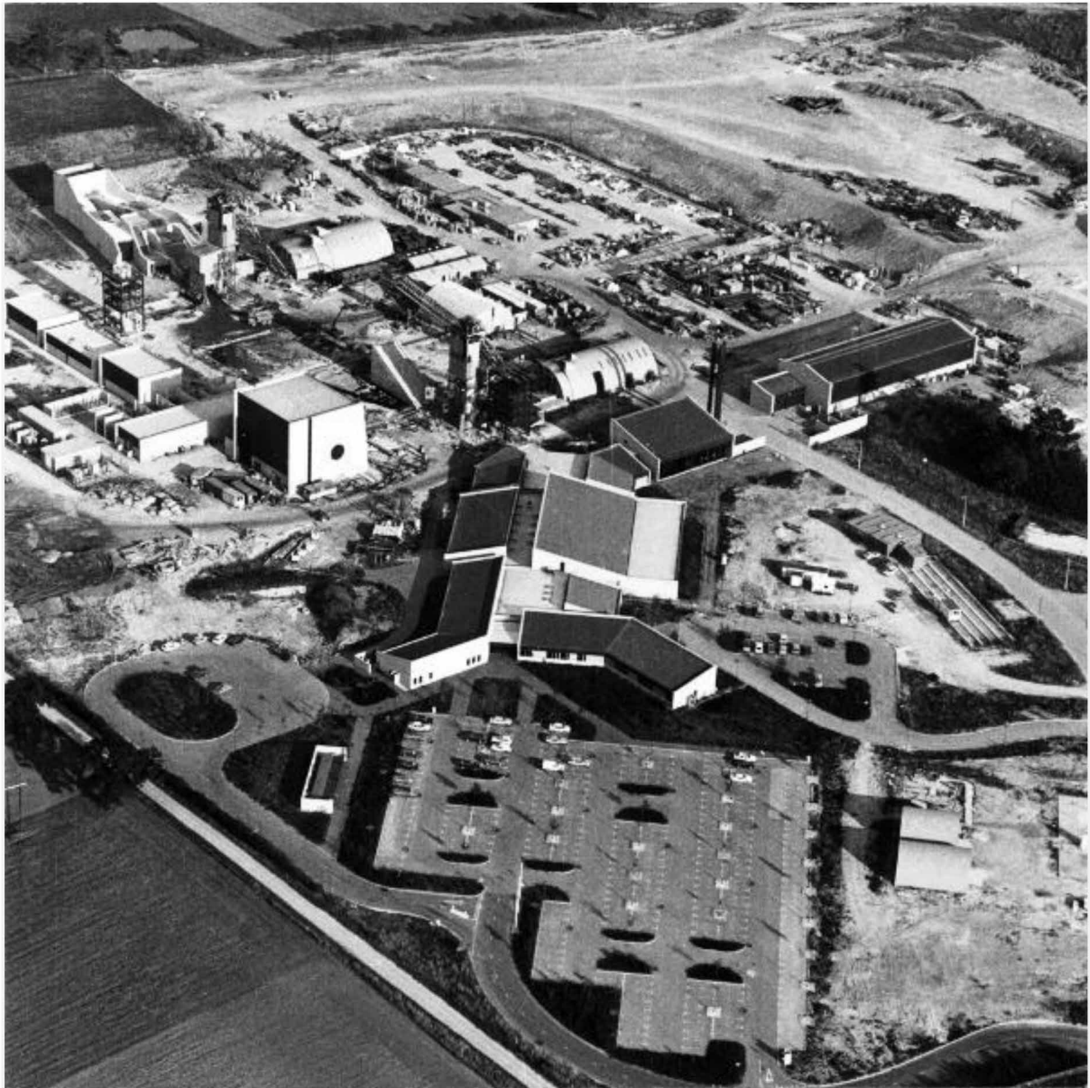
North Selby Mine 1985
