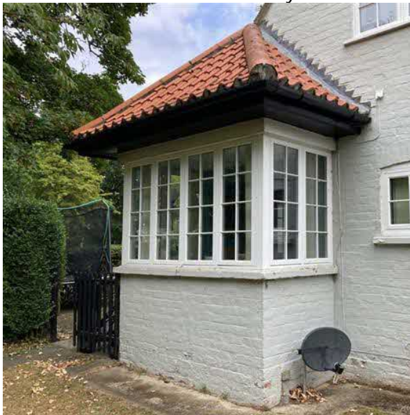
Rear view of bay
