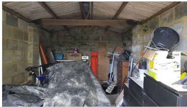
16. Interior of garage
