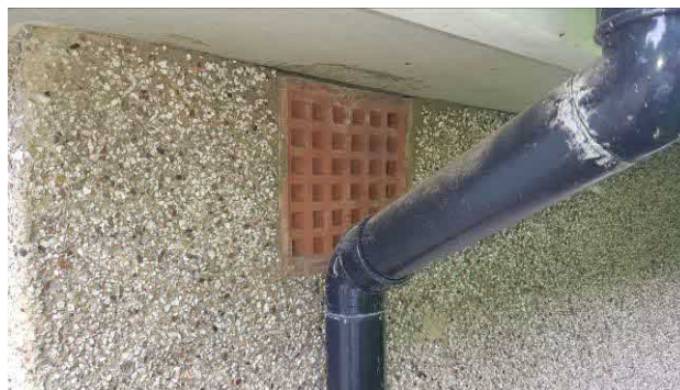
13. Vent hole in wall
