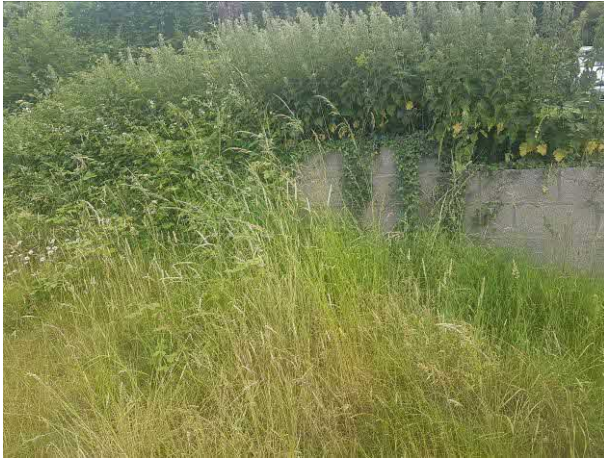
28. Breeze block wall proposed for removal
